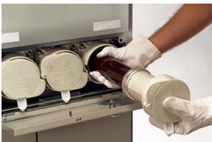
Removal of the fuse
