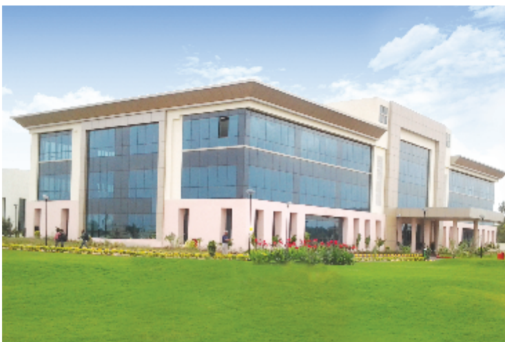
Switchgear Factory, Vadodara
