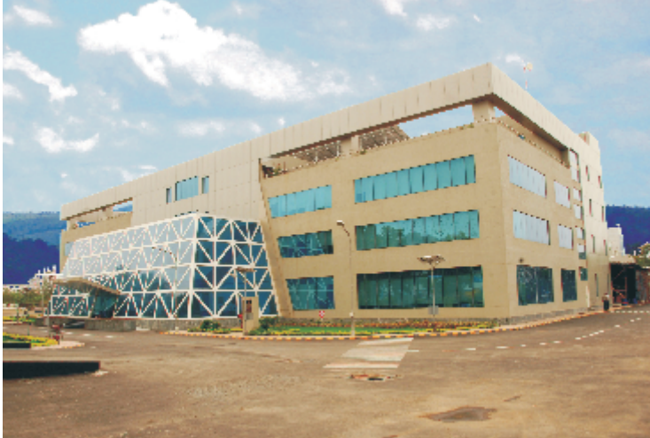
Switchgear Factory, Navi Mumbai
