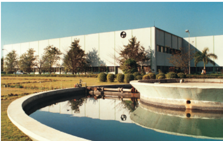
Switchgear Factory, Ahmednagar
