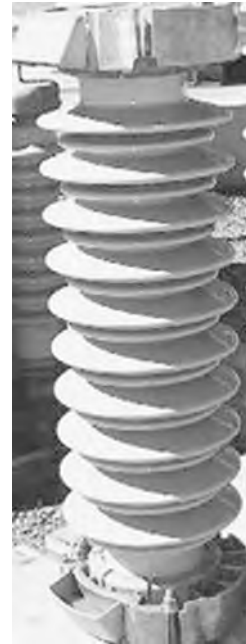
FIGURE 10.8 Post insulators.
