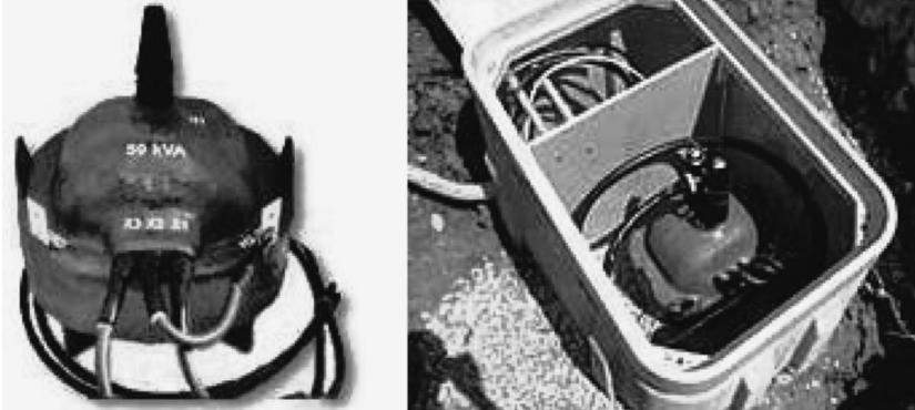
FIGURE 3.25 Solid-insulation distribution transformer. (By permission of ABB Inc., Quebec.)
