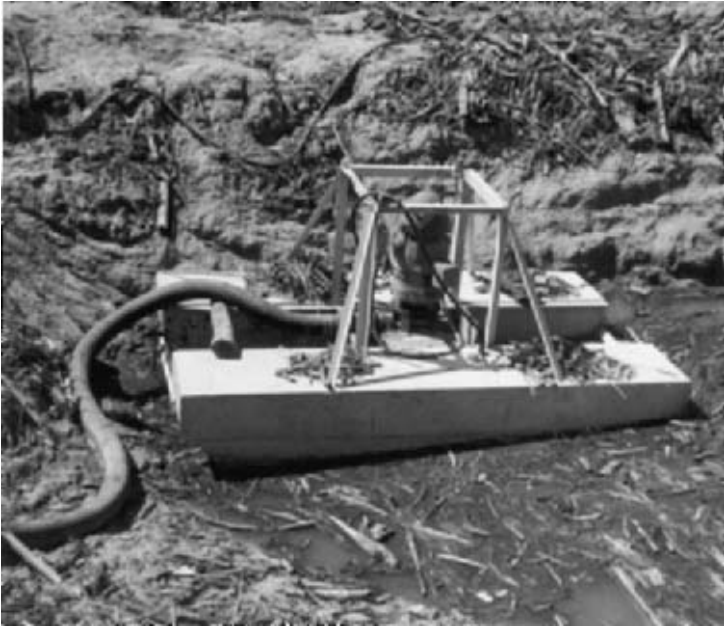
FIGURE 1 A simple barge (Hazleton Pumps, Inc.)
