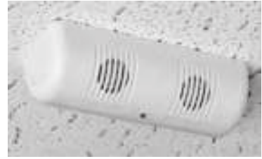
Figure 9.12.8. Ceiling occupancy sensor.
