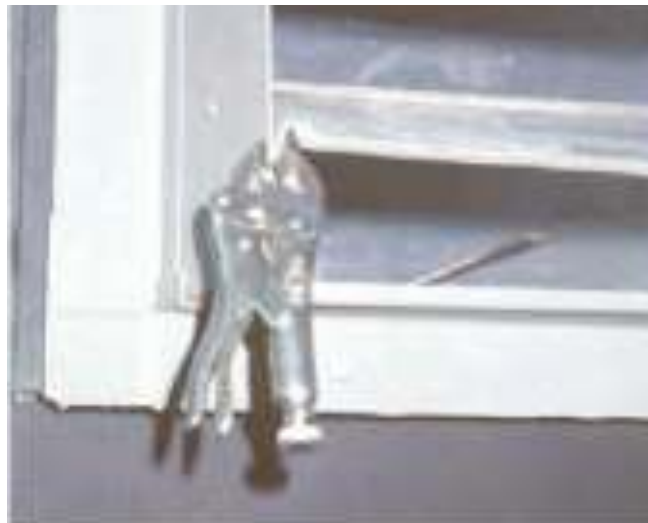
Figure 9.7.2. Damper quick fix – not recommended
