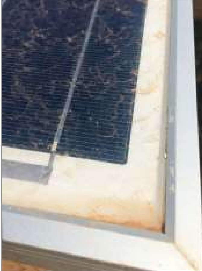
Figure 7. Module soiling can often be traced to a source, such as construction-site dust, resulting in about 5% loss. Photo by Andy Walker, NREL
