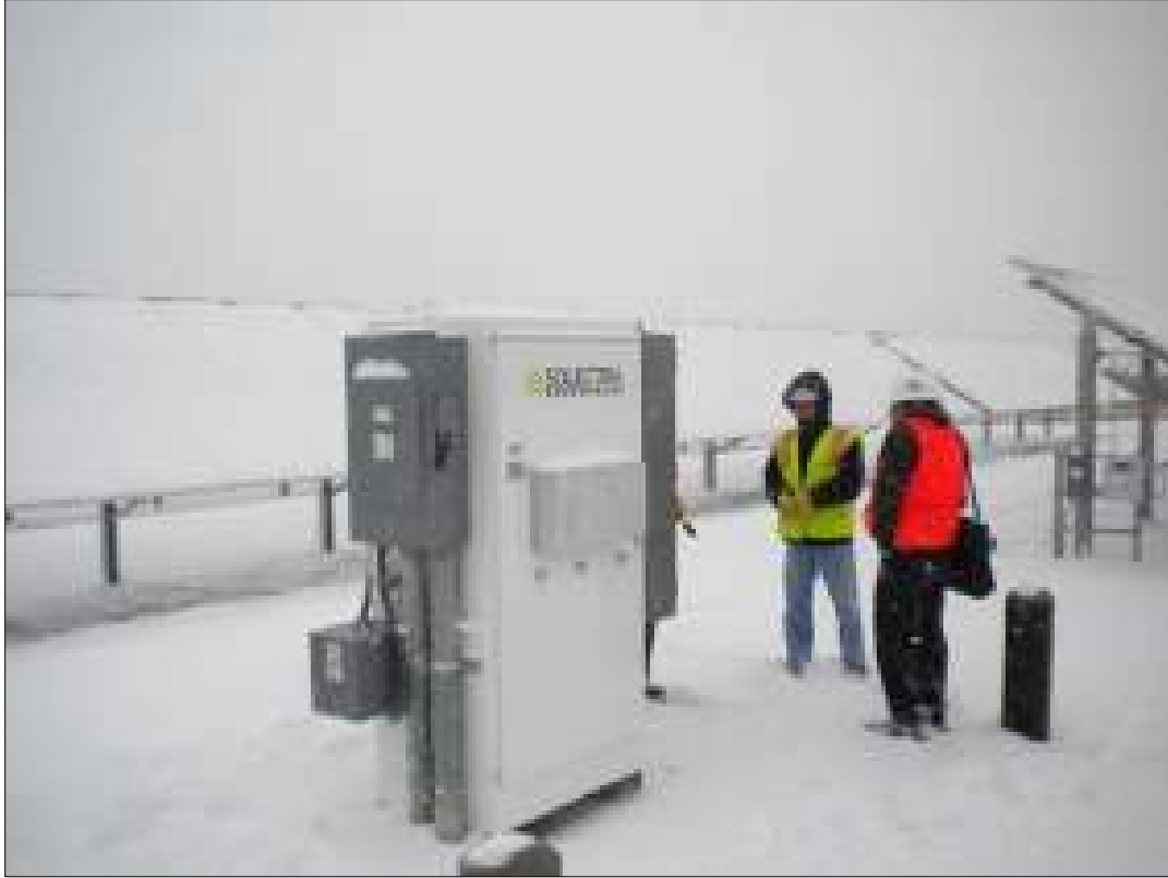
Figure 9. Snow is an environmental condition that both reduces performance and complicates provision of O&M services, but removal of snow off arrays is not recommended due to the potential for damage. Photo by Andy Walker, NREL
