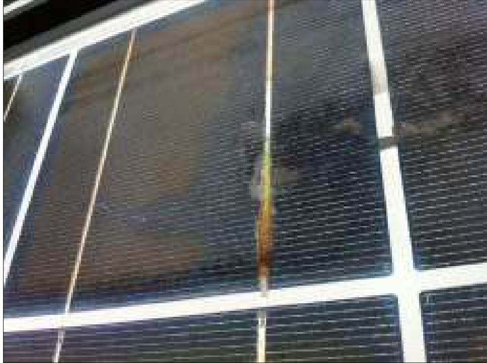
Figure 18. Cracked or peeling backsheet leads to water infiltration and ribbon corrosion. Photo by Andy Walker, NREL
