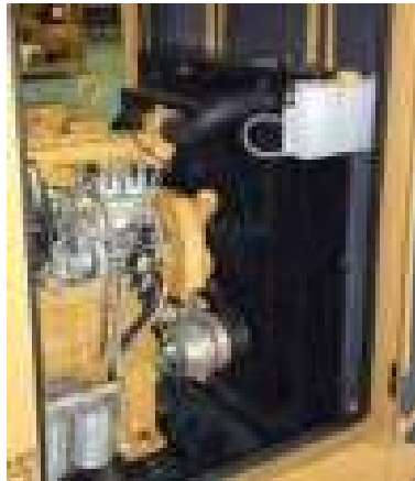
Fig. B1.4 Radiator Cooling System
