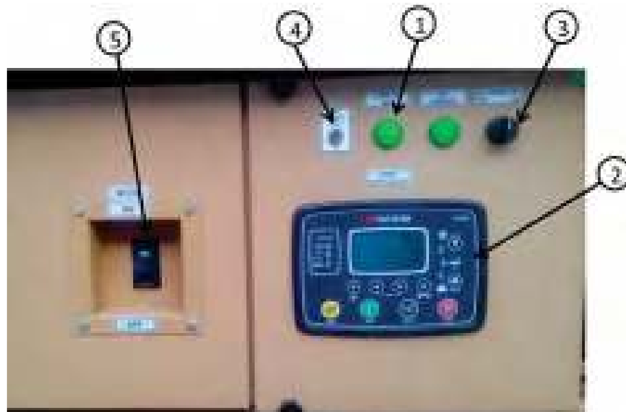
Fig. E5.0(a) Exterior Illustration of DATAKOM Control Panel & Power Panel
