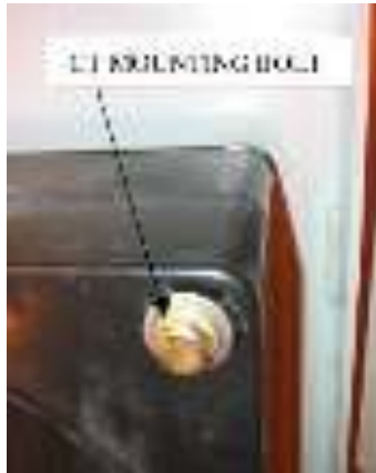
Figure 80. CT Mounting Bolt
