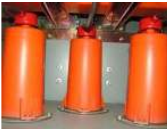
Figure 22. One Type of Metalclad Surge Suppressor
