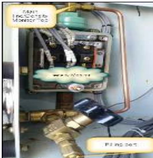
Figure 65. Filling Port on Manifold with Density Monitor
