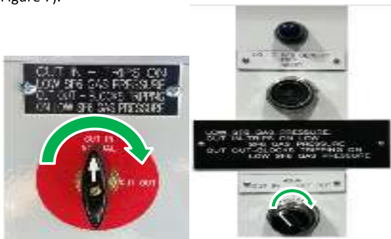
Figure 7. FCO, Lock Out Light and Reset Button
