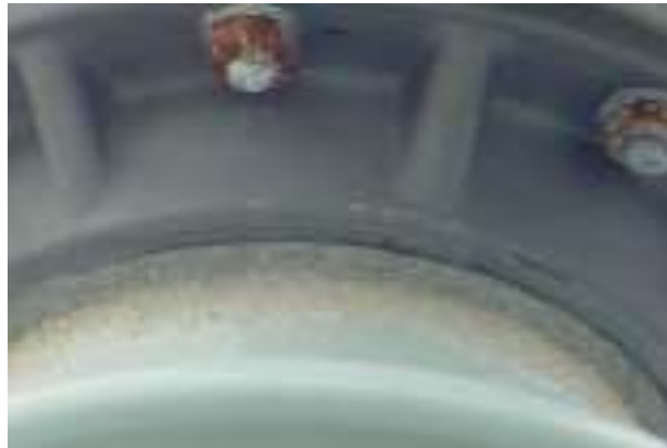
Figure 57. Possible Corrosion on Top Bushing Cap Hardware for Certain MEPPI SF 6 Breakers
