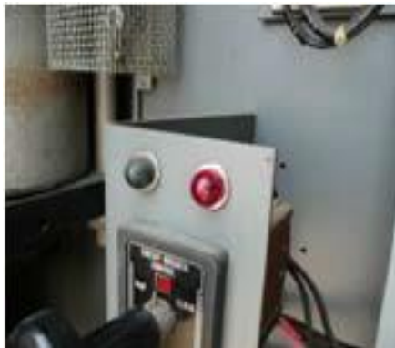
Figure 1. Typical Installation of a Receptacle Without a Resistor
