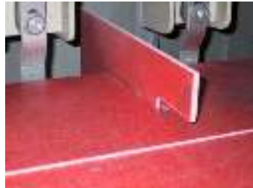
Metalclad Cell Without Corona
