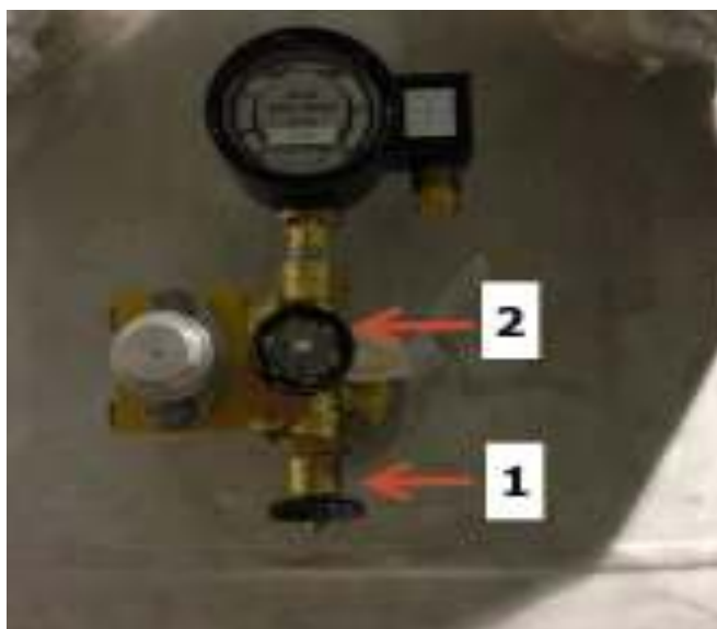
Figure 11. Hyoda Density Monitor with Dilo D20 Fill Port
