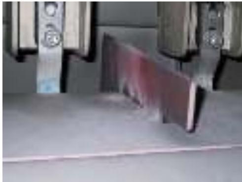
Metalclad Cell with Corona Activity
