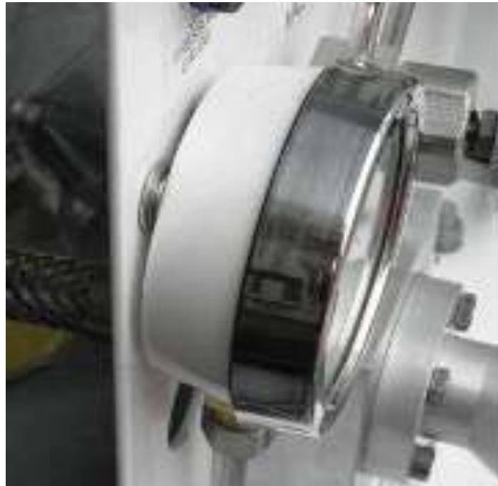
Figure 56. Faulty SF 6 Gauge with White Plastic Housing
