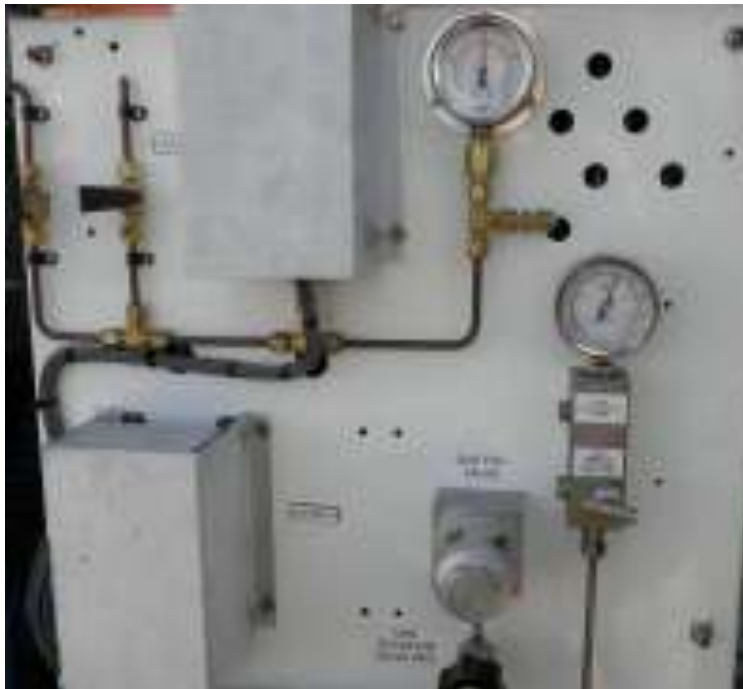
Figure 55. Location of Air Bleed Orifice on MEPPi 500 kV Breakers
