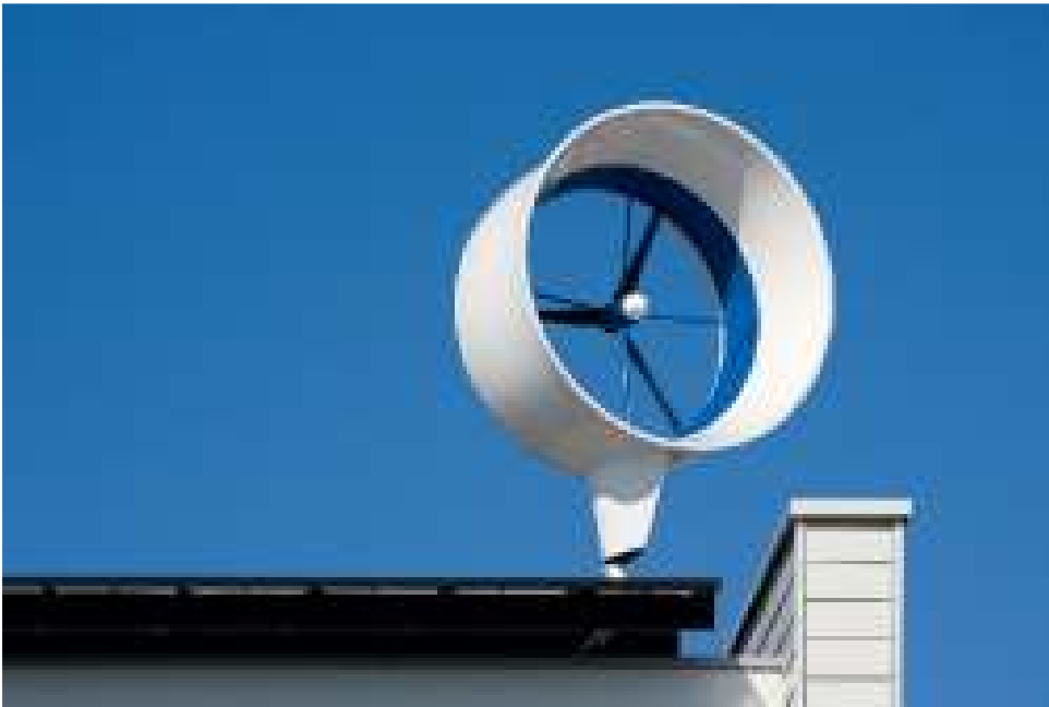
Figure 2.5 Small wind generator on a domestic property.
