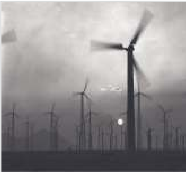
Figure 14.9 San Gorgino wind farm, Palm Springs, California, USA.
