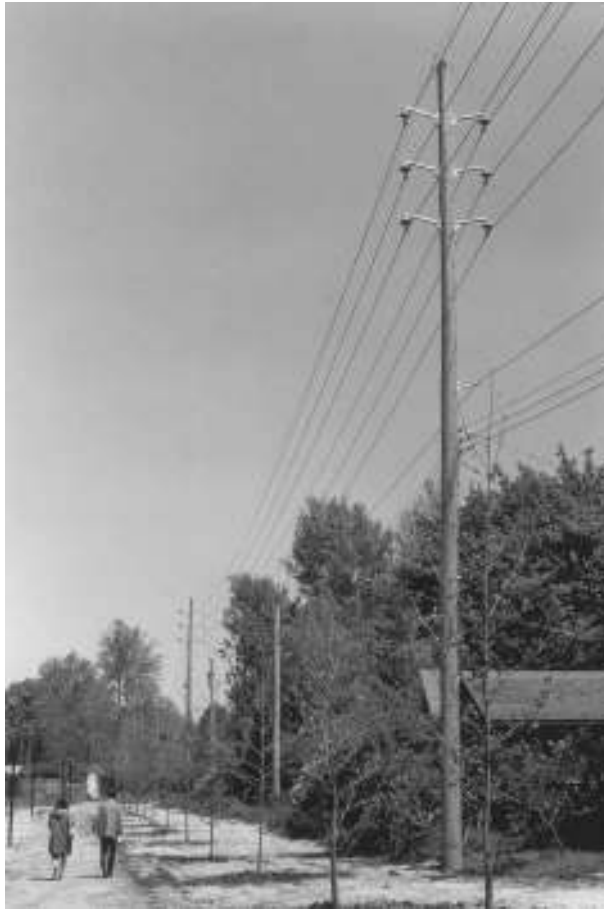
FIGURE 2.20 A typical 34.5-kV line with a double circuit and wood poles. It has a newer style construction. (Union Electric Company.)
