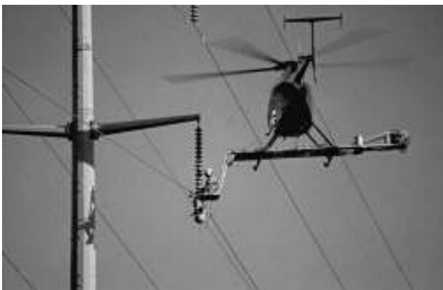
FIGURE 2.15 A lineman working from a helicopter platform.
