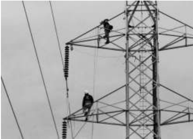
FIGURE 1.4 A transmission line that is being upgraded.
