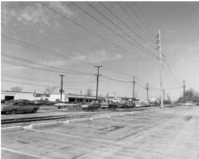
FIGURE 2.22 A typical 34.5-kV line with a double circuit and wood poles. It also has a 4.16-kV underbuild line and a 34.5-kV switch. (Union Electric Company.)
