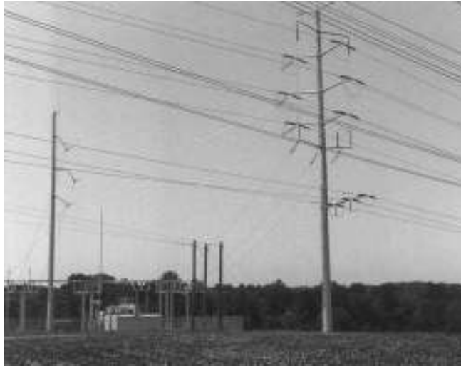
FIGURE 2.5 A double circuit 138-kV line built by using steel poles, having two 138-kV two top circuits and a 34.5-kV single circuit underbuild. (Union Electric Company.)
