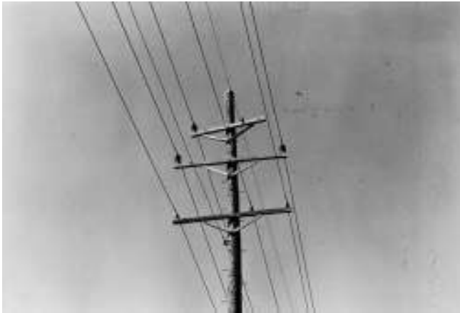
FIGURE 2.21 A 34.5-kV line with a single circuit and wood poles. It also has a 12.47-kV underbuild line and 34.5-kV switch. It has an old style construction. (Union Electric Company.)
