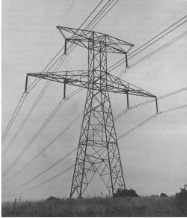
FIGURE 2.9 A typical 345-kV transmission line with bundled conductors and double circuit on steel towers. (Union Electric Company.)
