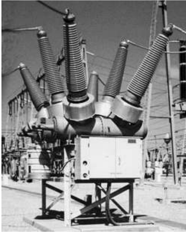
FIGURE 10.2 Three-pole-operated 245 kV SF 6 dead-tank circuit breaker fitted with 80-kA interrupters. (Courtesy of ABB Corporation.)
