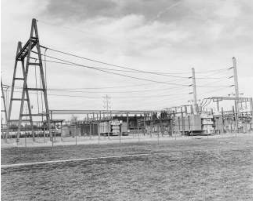
FIGURE 2.25 A bulk power substation operating 138/34.5-kV voltage level. (Union Electric Company.)
