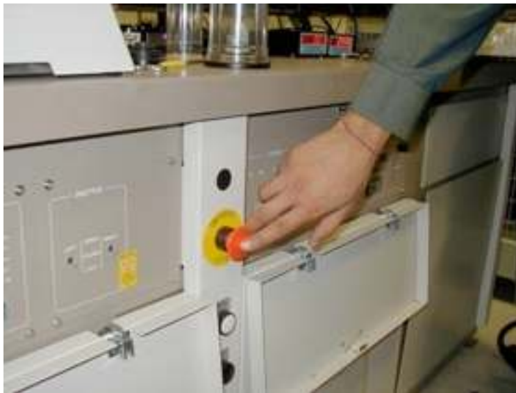
Fig. 5.3.1.b – An Emergency Stop (E-Stop) does not cut all electrical power to equipment.
