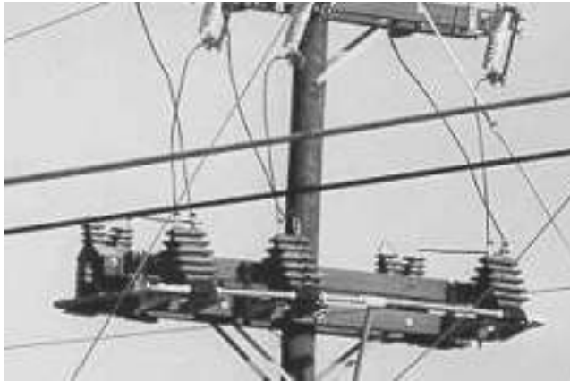
FIGURE 7.29 15-kV three-phase/four-wire metering rack with 3 VT and 3 CT. (Photo courtesy of Kuhlman Electric Corp.)
