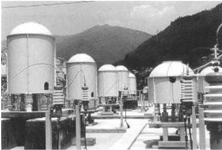
FIGURE 10.48 Installation of harmonic filter reactors for an HVDC project with a sound-shield enclosure.
