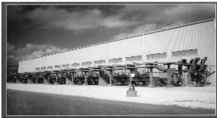
FIGURE 5.21 A 36-pulse system made up of 12 transformers with six types of six-pulse transformers for high-current electrochemical rectifier duty. Each transformer is 11,816-kVA OFWF with 426-V delta secondary windings. Each transformer has a 34,500-V primary with the shifts shown in Table 5.7 for a 36-pulse system. (Photo courtesy of Niagara Transformer Corp.)
