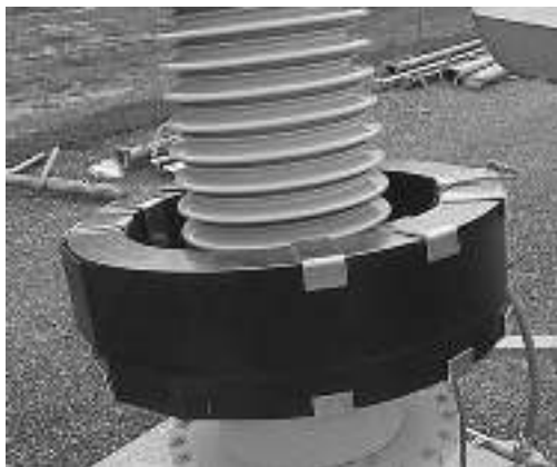
FIGURE 7.27 600-V-class slipover CT installed on high-voltage bushing with ground shield. Note the ground lead going back through the CT window to avoid shorted electrical turn. (Photo courtesy of Kuhlman Electric Corp.)
