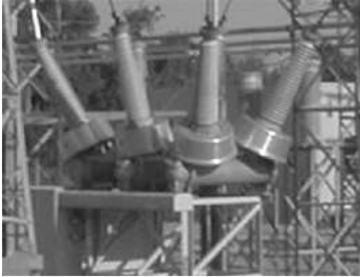
FIGURE 7.28 High-voltage circuit breaker with BCTs mounted underneath a metallic cover. (Photo courtesy of Kuhlman Electric Corp.)
