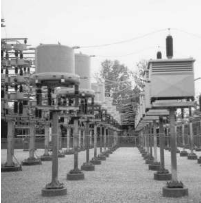
FIGURE 10.43 AC filter for an HVDC project; capacitors, tapped filter reactors, and separately mounted resistors.
