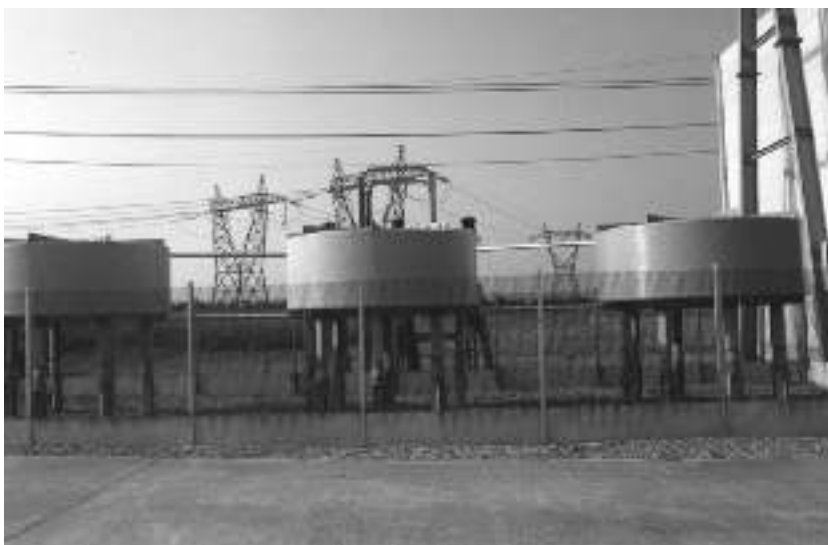
FIGURE 10.25 20 kV, 20 MVA (per phase) tertiary connection shunt reactors.
