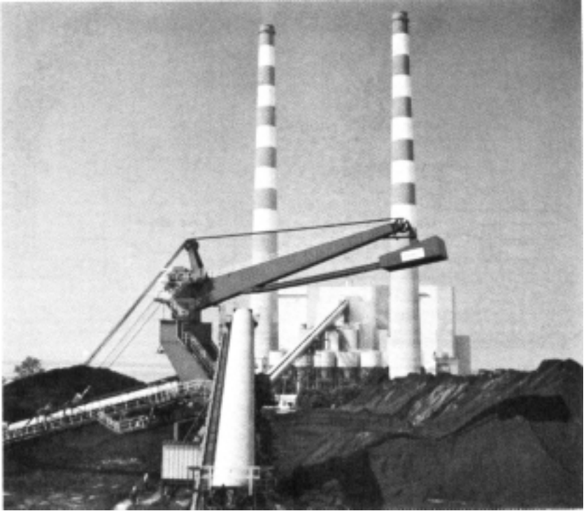
Figure 3-1. Coal Pile ( Courtesy LILCO )
