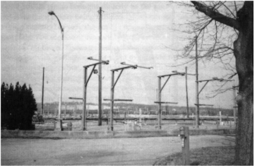
Figure 3-4. Buried Gas Tanks ( Courtesy LILCO )
