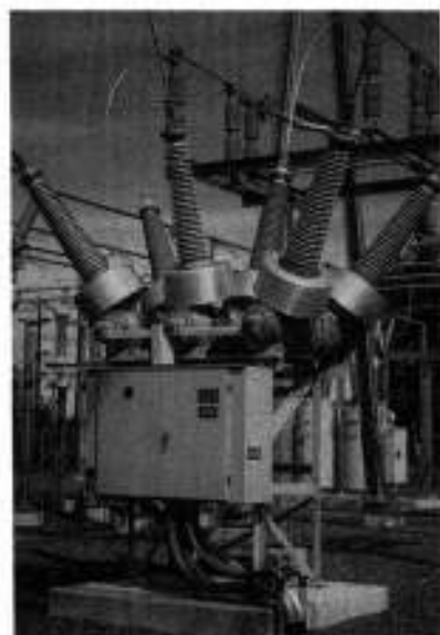
Figure 5.34 Dead tank puffer type circuit breaker ABB Power T&D.
