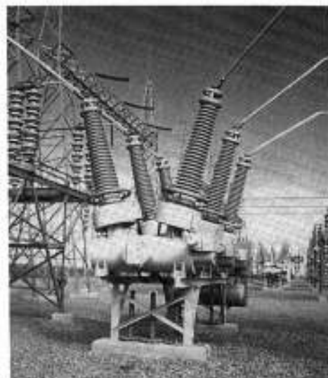
Figure 5.3 Dead tank type circuit breaker (grounded enclosure).
