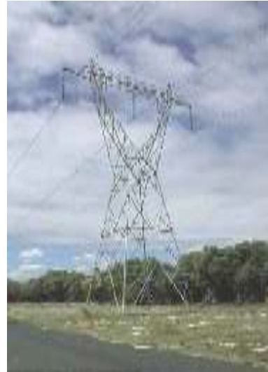
Fig. 5.16: High voltage line with two overhead screen wires
