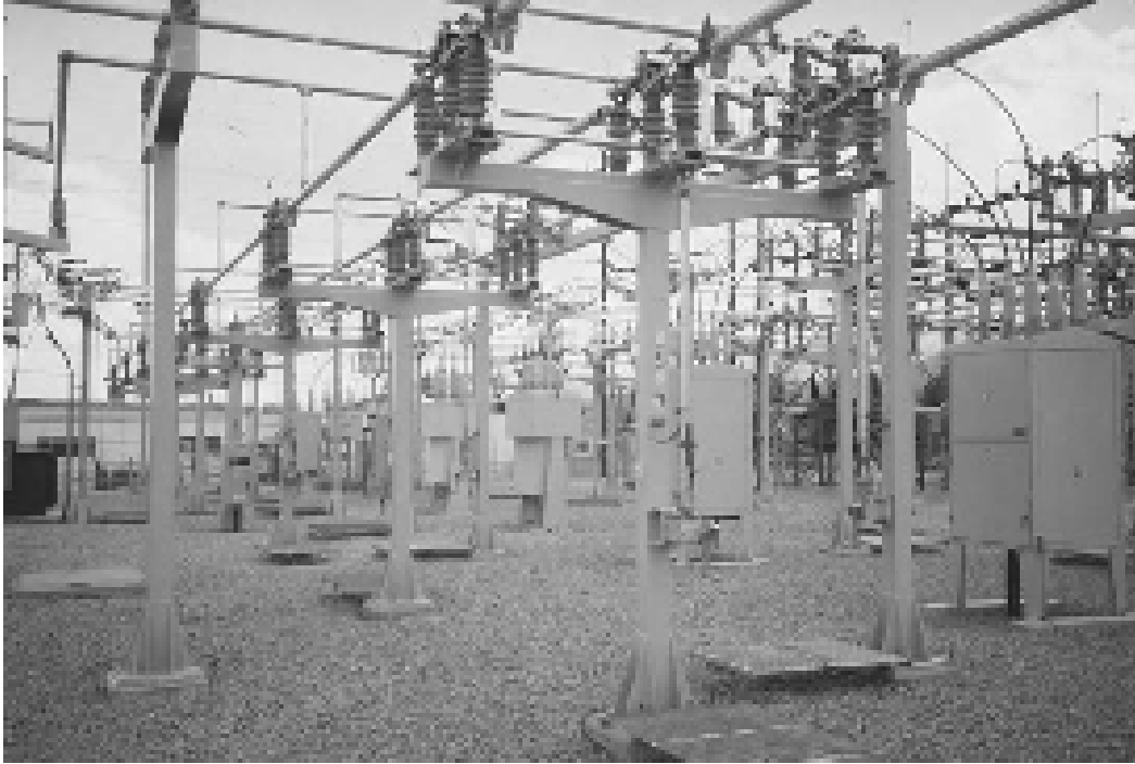
Figure 4-38. Examples of a typical electrical bus.
