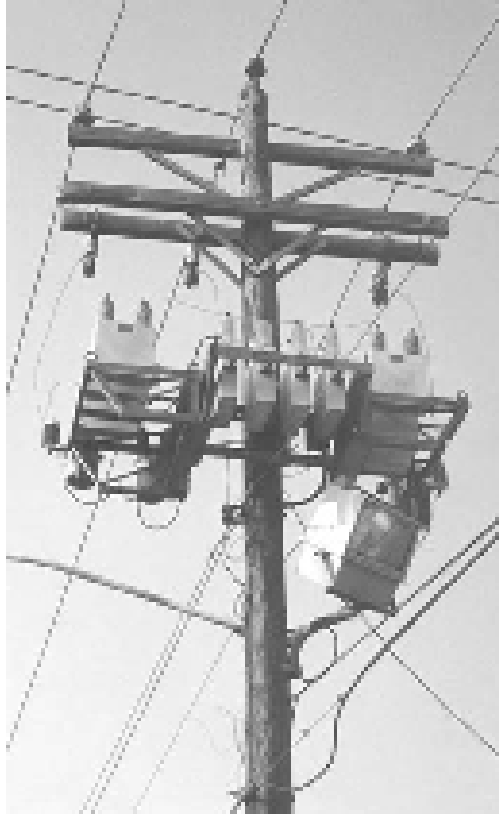
Figure 4-40. Distribution capacitor bank.
