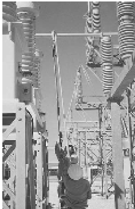
Figure 10-8. Live maintenance on transmission lines.
