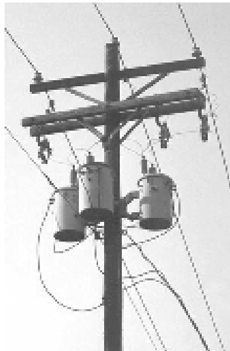
Figure 5-18. Three-phase transformer bank.
