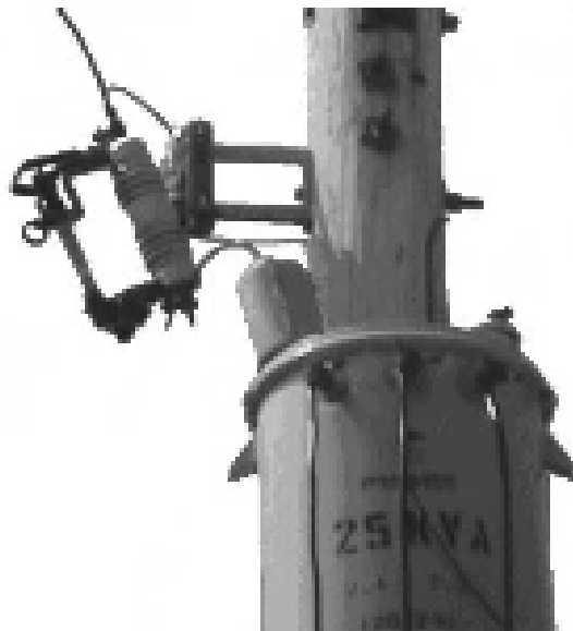
Figure 5.24. Distribution fuses.
