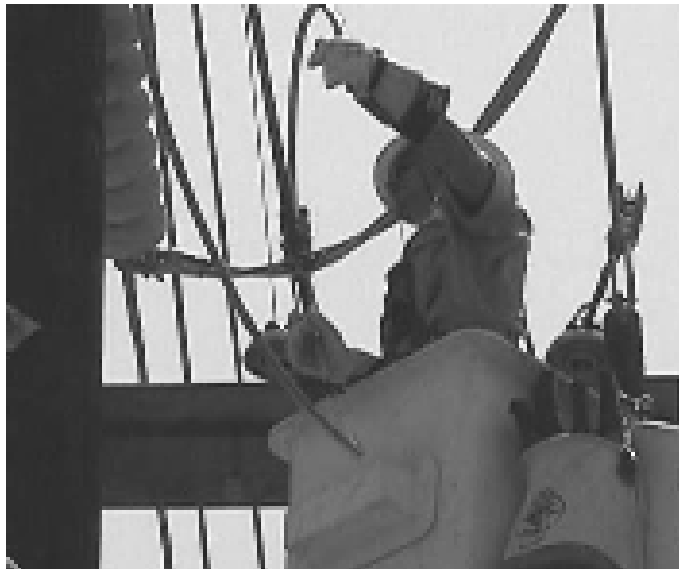
Figure 10-11. Live maintenance distribution. Courtesy of Alliant Energy.
