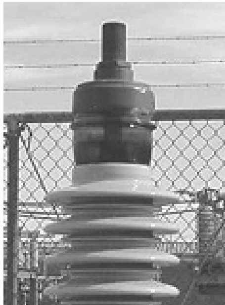
Figure 4-7. Bushing oil level gauge.
