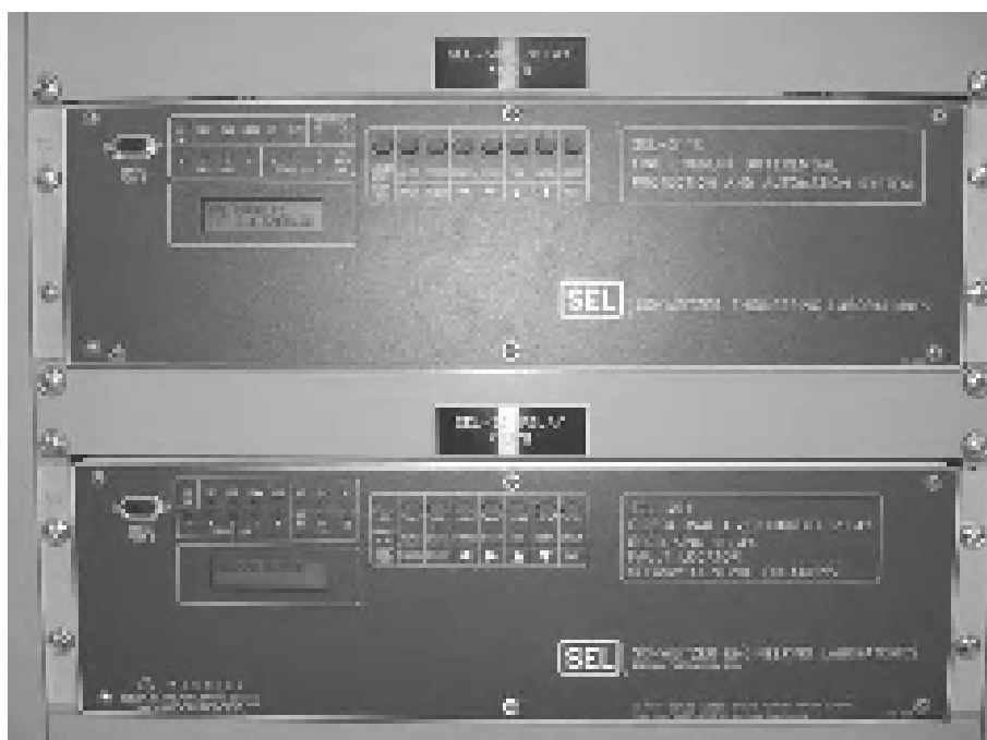
Figure 7-1. Solid-state relays.
