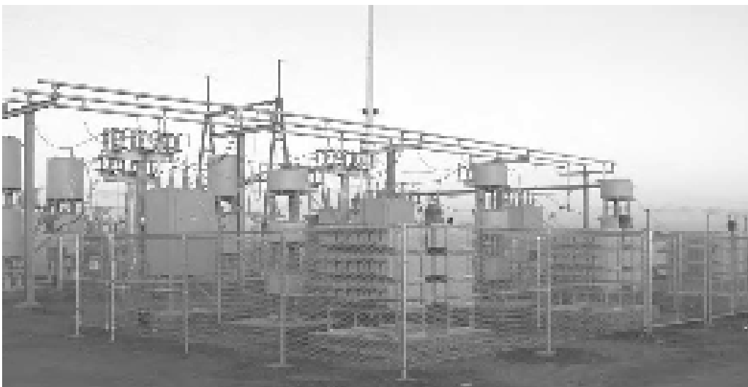
Figure 4-42. Static VAR compensator. Courtesy of Jeff Selman.
