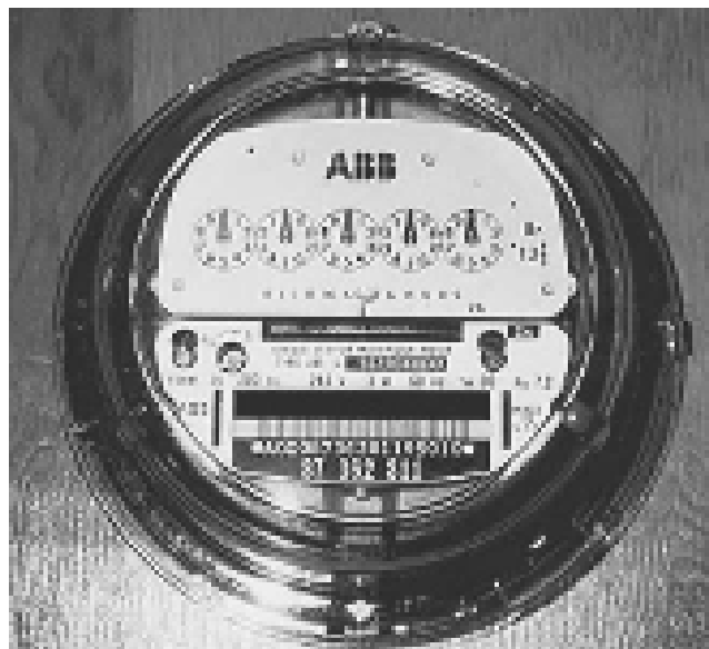
Figure 6-6. Electromechanical kWh meter.
