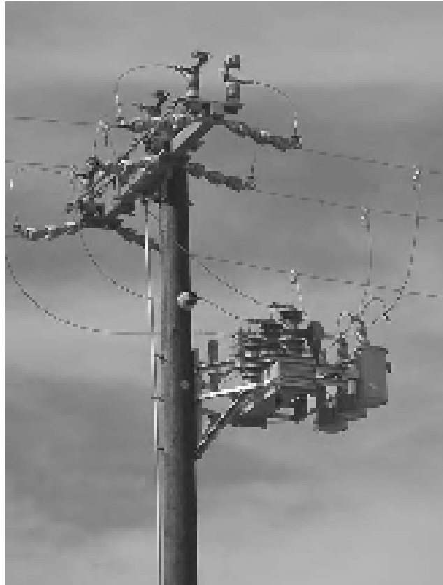
Figure 6-11. Overhead primary metering.
