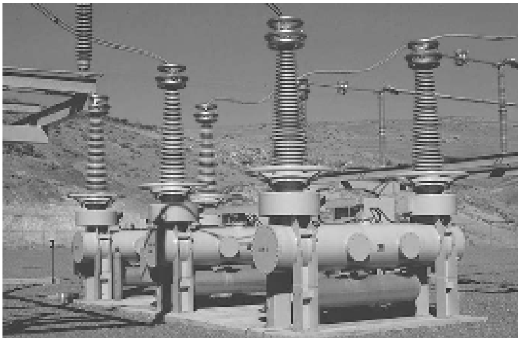
Figure 4-26. 345 kV Gas breaker.
