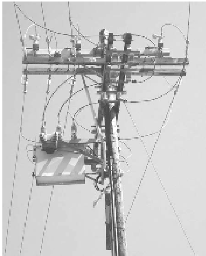
Figure 4-30. Distribution line recloser. Courtesy of Alliant Energy.
