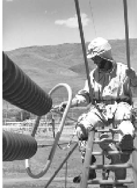
Figure 10-9. Bare-hand, live-line maintenance.
