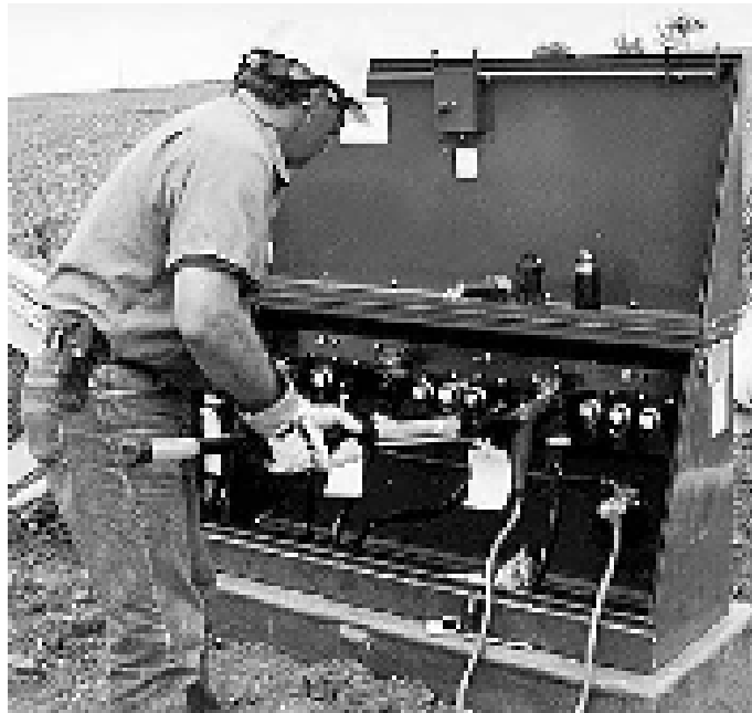
Figure 5-29. Load-break connections. Courtesy of Alliant Energy.
