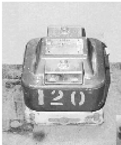
Figure 4-13. Low-voltage PT. Courtesy Alliant Energy.
