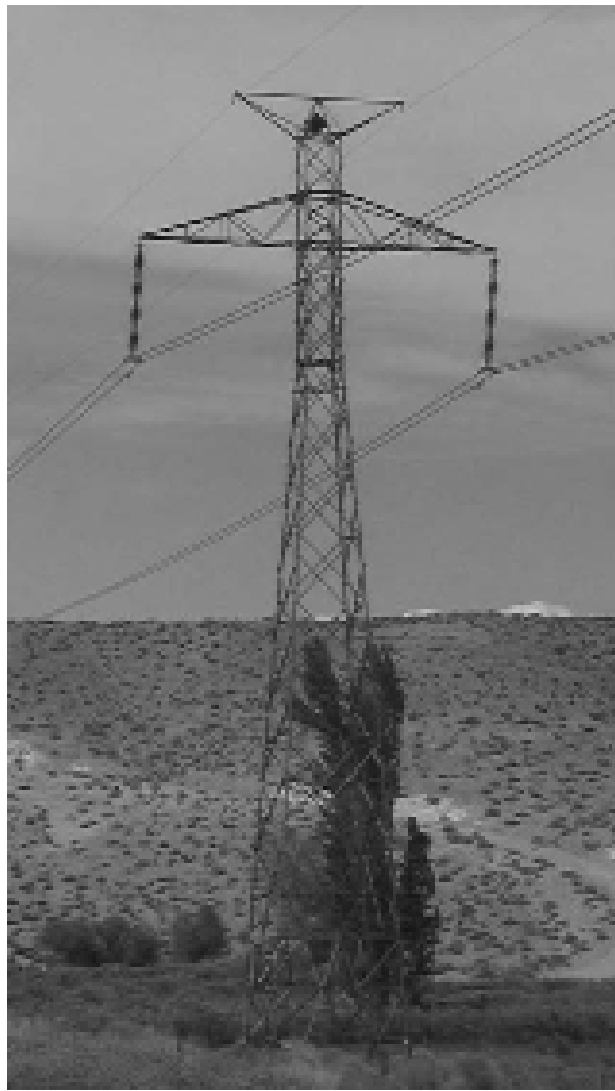
Figure 3-7. Overhead dc transmission line.
