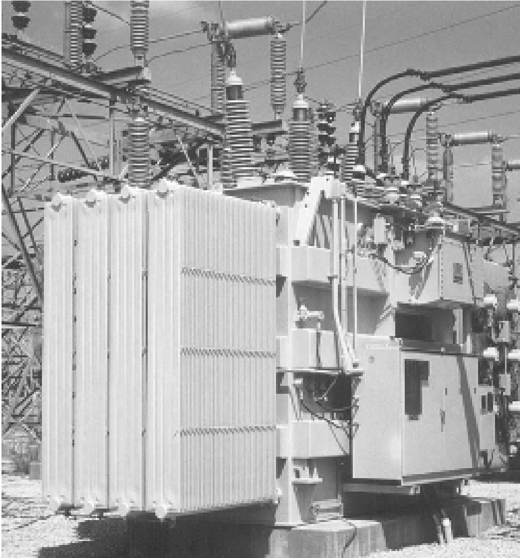
Figure 4-2. Distribution power transformer.
