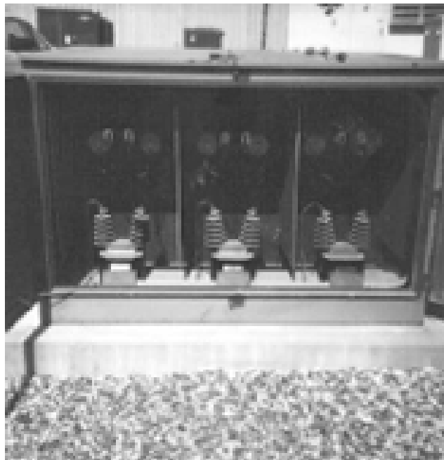
Figure 6-10. Underground primary metering. Courtesy of Alliant Energy.
