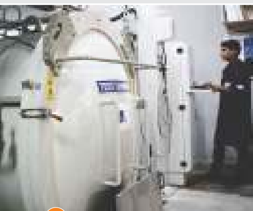
SF6 Insulated Indoor Ring Main Unit
