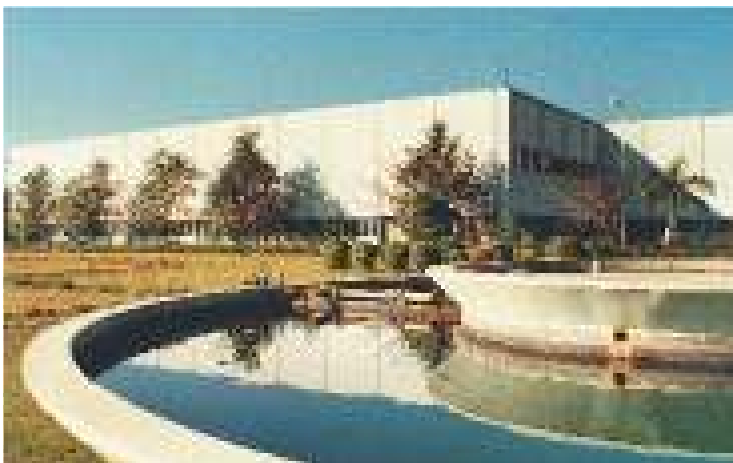
Switchgear Factory, Ahmednagar
