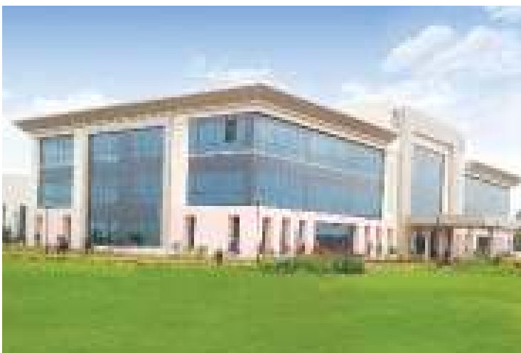
Switchgear Factory, Vadodara
