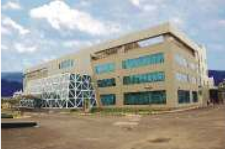
Switchgear Factory, Navi Mumbai
