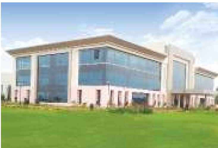
Switchgear Factory, Vadodara
