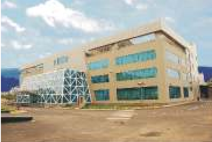
Switchgear Factory, Navi Mumbai
