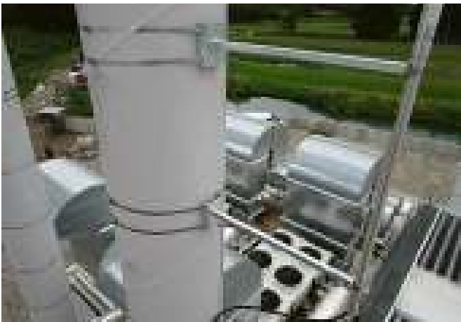
Spacer with tensioning strap fastener
