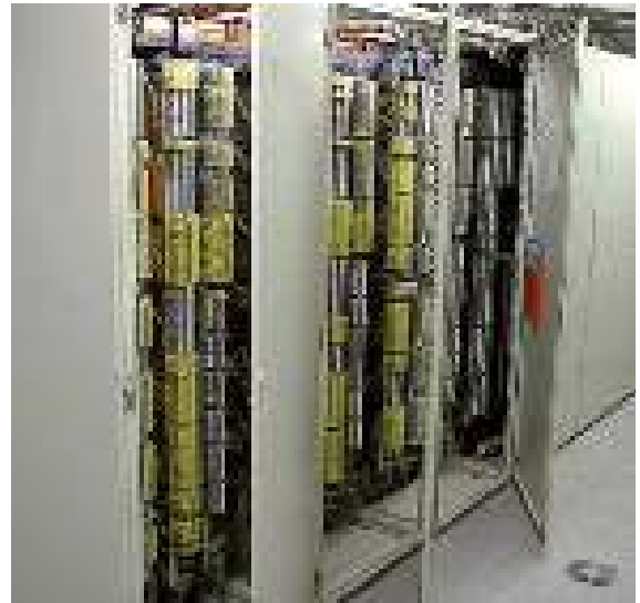
Figure 9.4.6 DEHNconnect terminal blocks with integrated surge protection for protecting the complete measuring and control equipment
