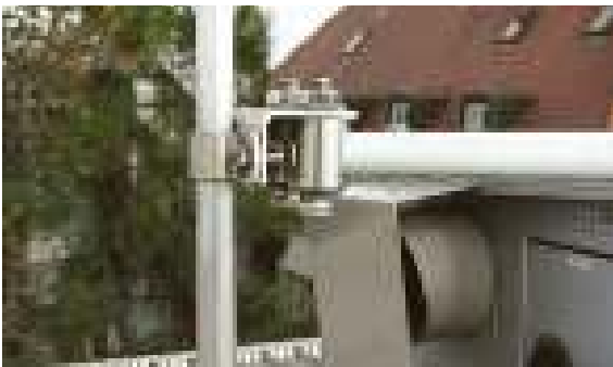
Figure 5.1.8.5 Supporting element for an air-termination rod
