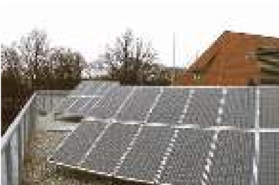
Figure 5.1.8.6 Isolated air-termination system of a photovoltaic system
