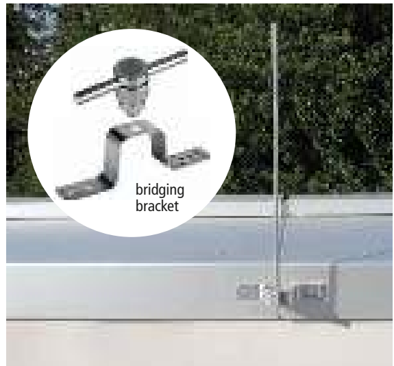
Figure 5.1.3.4 Example how to protect the metal capping of the roof parapet if melting is not allowed (front view)
