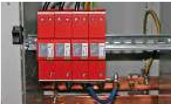
Figure 9.16.8 Coordinated type 1 surge arrester
