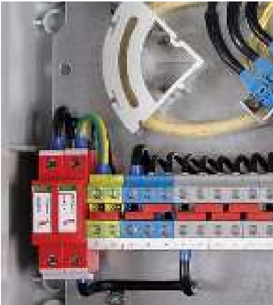
Figure 9.17.6 Prewired hybrid box for 48 V d.c. outdoor installations with DEHNguard type 2 arrester
