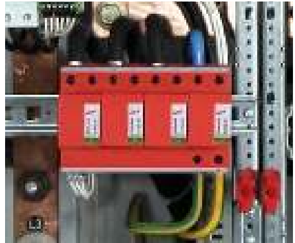
Figure 7.5.2.7 DEHNventil combined arrester
