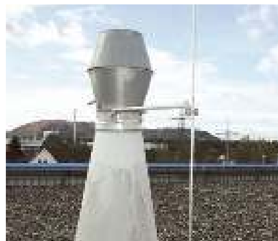
Figure 5.1.8.3 Air-termination rod with spacer
