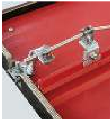
Figure 5.1.4.6 Sample construction on a standing seam roof
