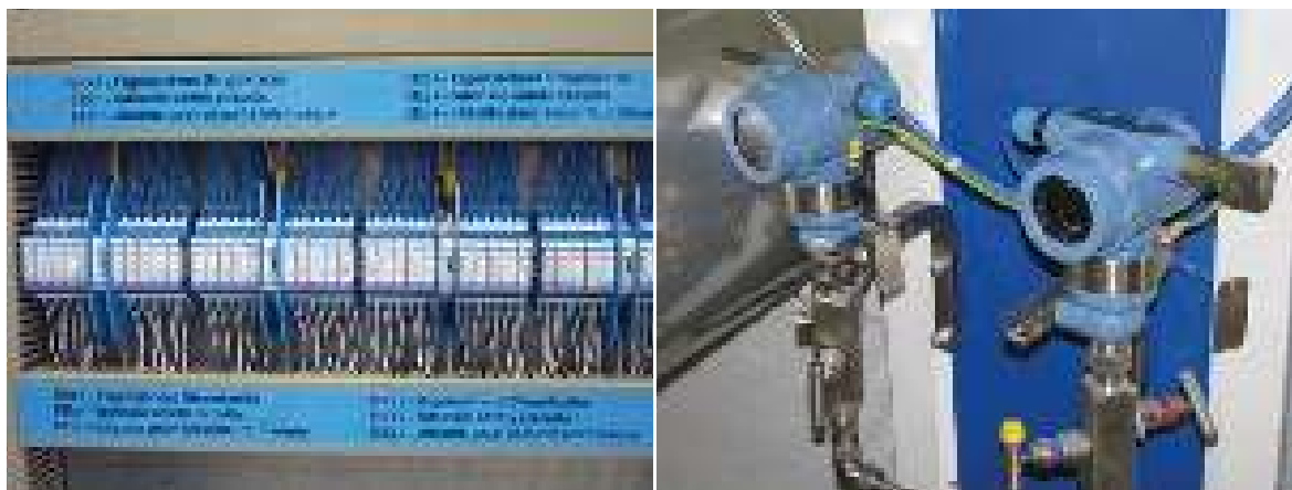
Figure 9.32.5 Surge protective devices for intrinsically safe measuring circuits
