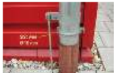
Figure 5.2.2.1.4 Earth connection of a downpipe
