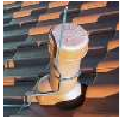
Figure 5.1.2.3 Additional air-termination system for vent pipes
