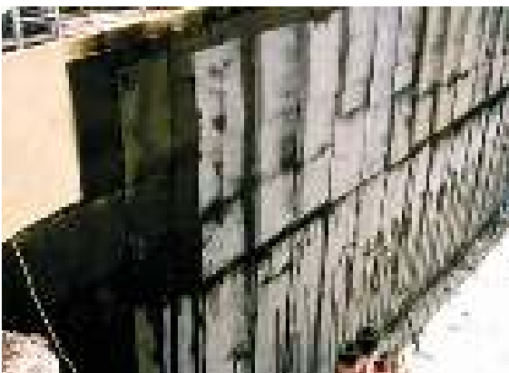
Figure 5.5.2.18 Bituminous sheetings used as sealing material
