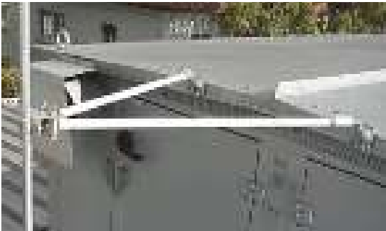
Figure 5.1.8.4 Angled support for an air-termination rod
