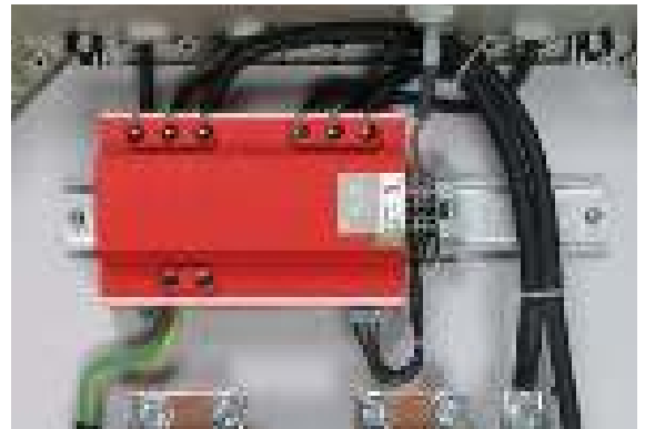
Figure 9.18.8 DEHNlimit PV 1000 V2 spark-gap-based type 1 combined arrester
