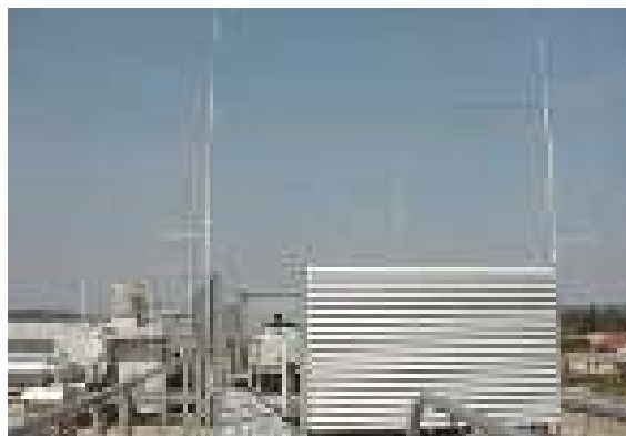
Figure 5.1.8.11 Isolated air-termination system with DEHNiso Combi
