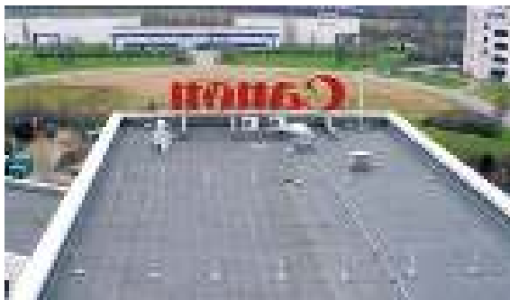
Figure 5.1.8.9 Elevated air-termination system; source: Blitzschutz Wettingfeld, Krefeld
