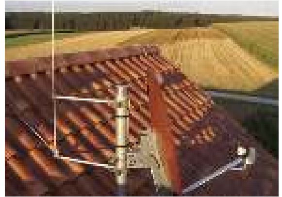
Figure 5.1.2.5 Antenna with air-termination rod and spacer
