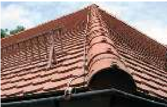
Figure 5.1.1.18 Gable roof with conductor holder
