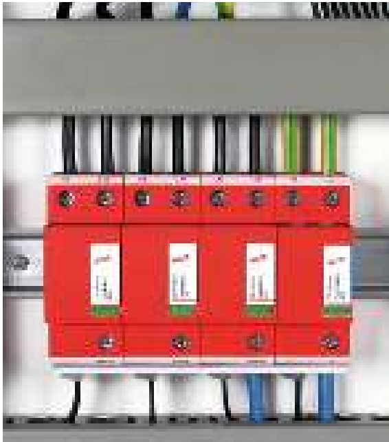
Figure 6.2.1 DEHNbloc M for installation in conformity with the lightning protection zone concept at the boundaries from O_A-1
