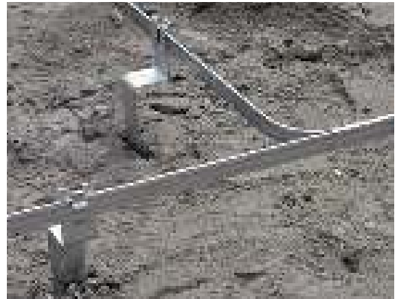
Figure 5.5.2.3 Foundation earth electrode
