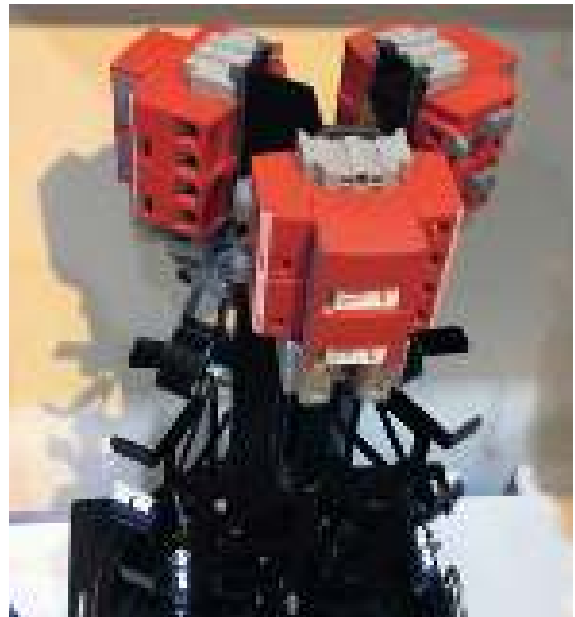
Figure 9.17.5 RRH installation protected by a type 1 arrester in a typical installation environment
