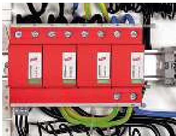
Figure 7.8.1.3 Modular DEHNventil M TNS combined arrester
