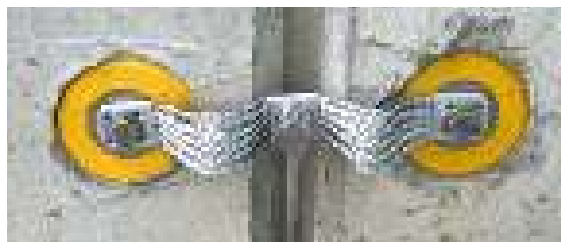
Figure 5.5.2.8 Bridging braid with fixed earthing terminals
