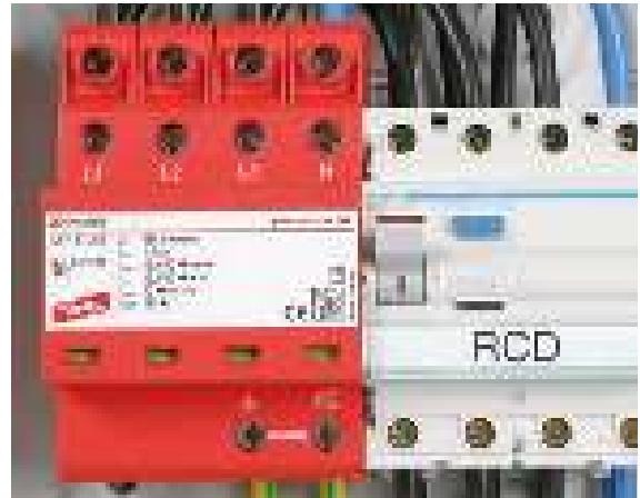
Figure 9.30.1 Prewired and application-optimised DEHNshield combined arrester with spark gap technology
