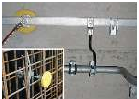
Figure 5.5.2.5 Fixed earthing terminal
