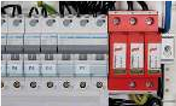
Figure 9.16.6 Modular type 2 surge arrester for protecting the 230/400 V supply
