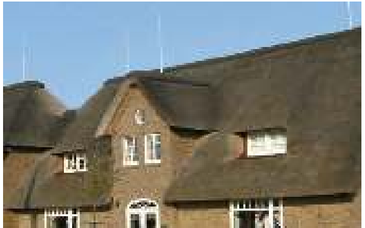
Figure 5.1.5.4 Historical farmhouse with external lightning protection system; source: Hans Thormählen GmbH & Co.KG.
