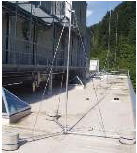
Figure 5.1.8.7 Isolated air-termination system for roof-mounted structures
