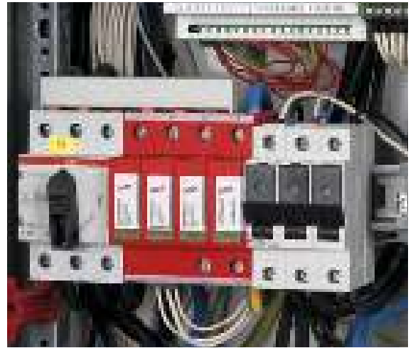
Figure 8.1.6.6 DEHNGuard modular CI: Type 2 surge arrester with integrated backup fuse
