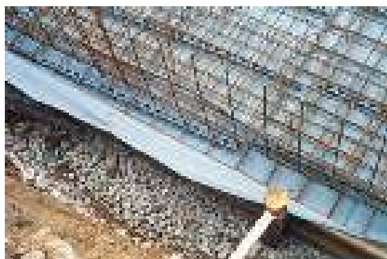
Figure 5.5.2.10 Membrane of foundation slabs
