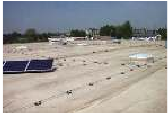
Figure 5.1.3.2 Practical use of air-termination rods
