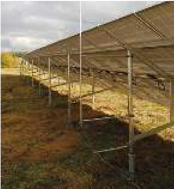
Figure 9.19.2 Lightning protection by means of DEHNiso spacers
