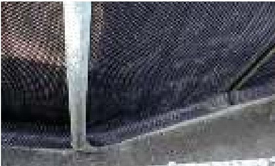
Figure 5.5.2.11 Use of dimpled membranes
