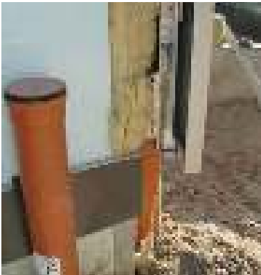
Figure 5.2.2.2.3 Earth connection of a metal façade
