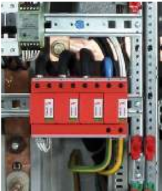
Figure 6.2.2 DEHNventil combined arrester for installation in conformity with the lightning protection zone concept at the boundaries from O_A-2
