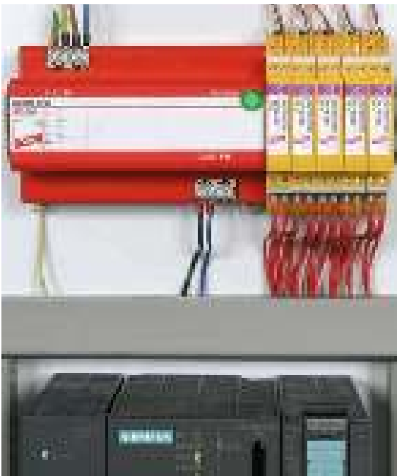
Figure 7.7.3.1 Protection of industrial electronic equipment (e.g. a PLC) by BLITZDUCTOR XT and SPS Protector
