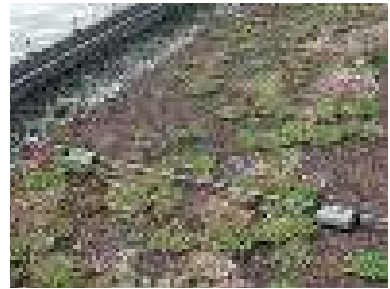
Figure 5.1.7.3 Conductor routing above the cover layer
