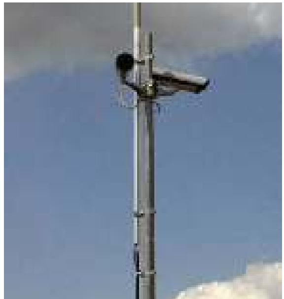
Figure 9.22.4 HVI Conductor installed at a pylon
