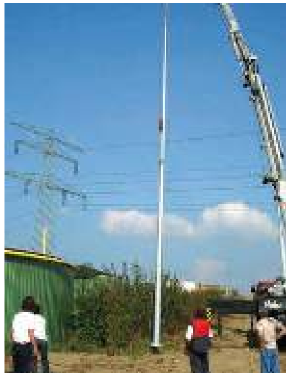
Figure 5.1.8.8 Installation of a telescopic lightning protection mast
