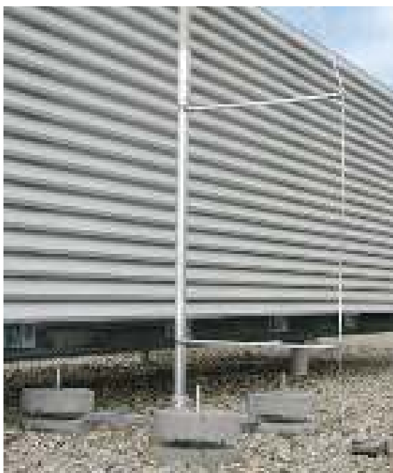
Figure 5.1.8.10 Tripod for isolated supporting tubes
