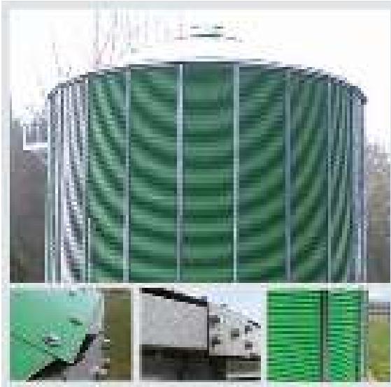
Figure 9.3.6 Fermenter made of bolted metal sheets
