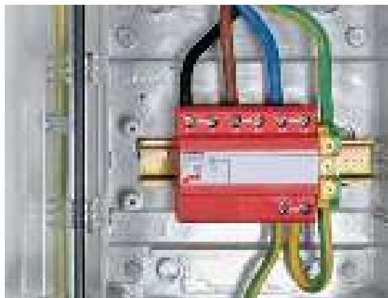
Figure 7.8.1.1 Three-pole DEHNBloc lightning current arrester
