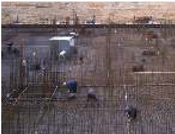
Figure 5.5.2.6 Meshed foundation earth electrode
