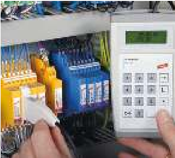
Figure 9.3.12 Combined arrester modules with LifeCheck
