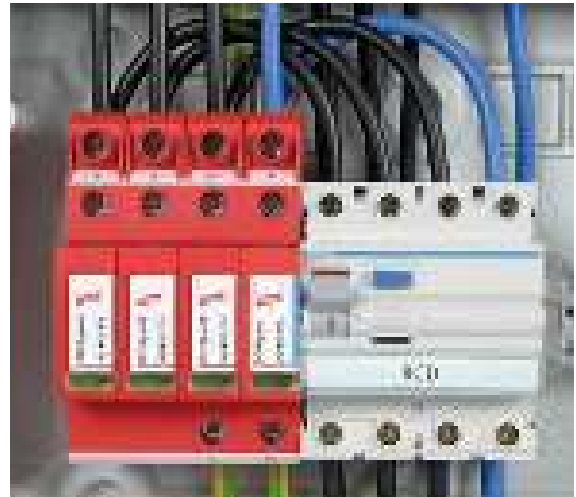
Figure 7.7.2.3 Multipole DEHNguard M TT surge arrester
