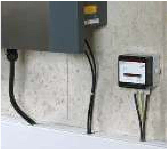
Figure 9.18.16 DEHNcube YPV SCI 1000 1M type 2 arrester for protecting inverters (1 MPPT)
