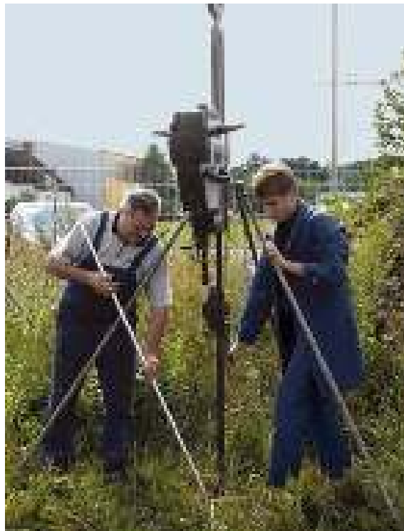
Figure 5.5.4.2 Driving an earth rod into the ground by means of a hammer frame and a vibration hammer
