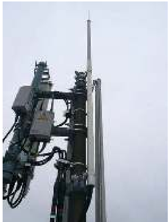
Figure 5.2.4.14 HVI Conductor installed on a radio tower
