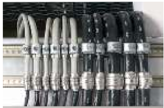
Figure 6.3.4 Lightning current carrying shield connection system (SAK)
