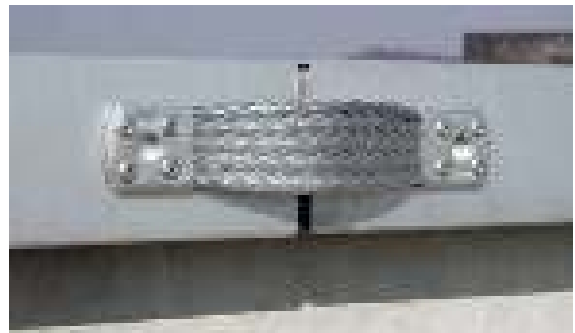
Figure 5.1.3.3 Bridging braid used for the roof parapet
