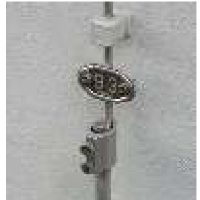
Figure 5.2.2.3.1 Test joint with number plate along a downpipe
