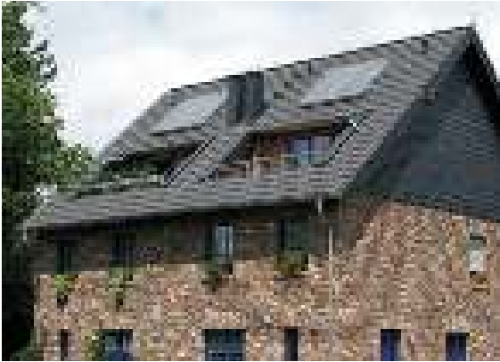
Figure 5.1.2.4 Building with photovoltaic system and sufficient separation distance; source: Blitzschutz Wettingfeld, Krefeld
