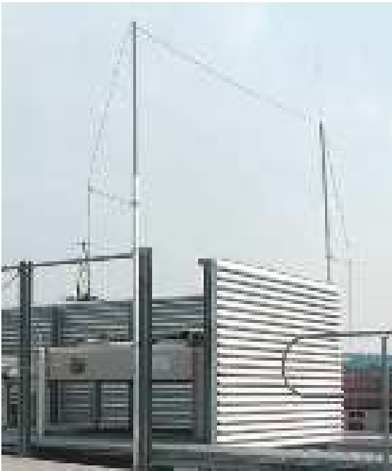
Figure 5.1.8.13 Isolated air-termination system with DEHNiso Combi
