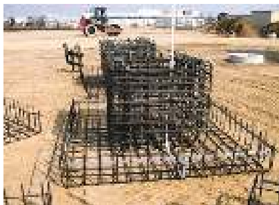
Figure 5.5.2.24 Foundation earth electrode for pad foundations with terminal lug; source: Wettingfeld, Krefeld
