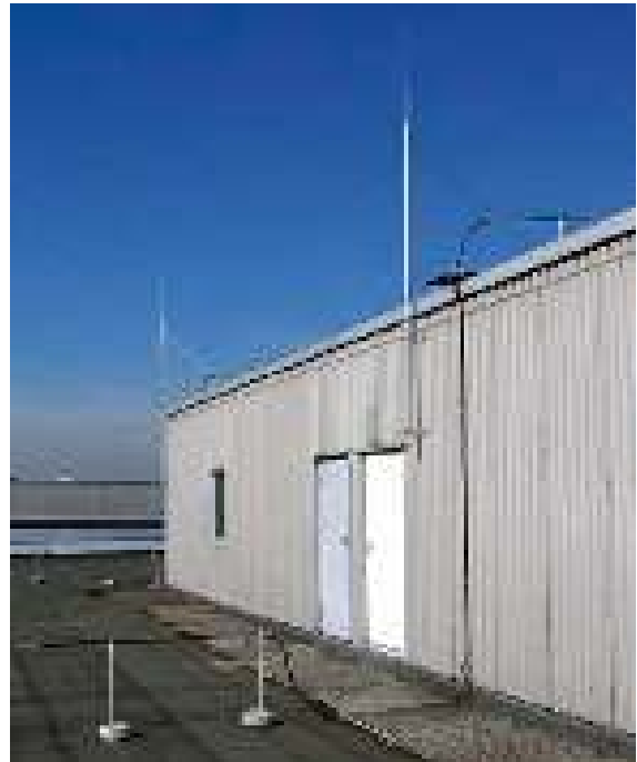
Figure 5.2.4.9 Installation of a HVI Conductor III with sealing end
