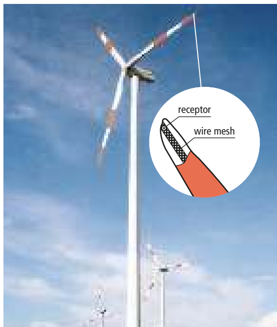
Figure 5.1.10.1 Wind turbine with integrated receptors in the rotor blades
