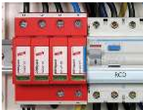
Figure 7.8.1.2 Multipole DEHNGuard M TT surge arrester
