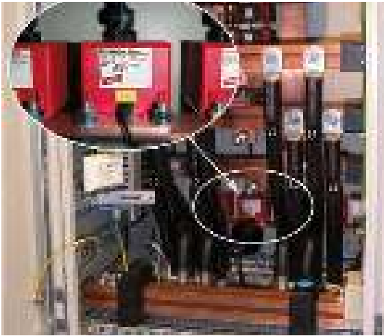
Figure 8.1.6.5 DEHNbloc Maxi S: Coordinated lightning current arrester with integrated backup fuse for busbars
