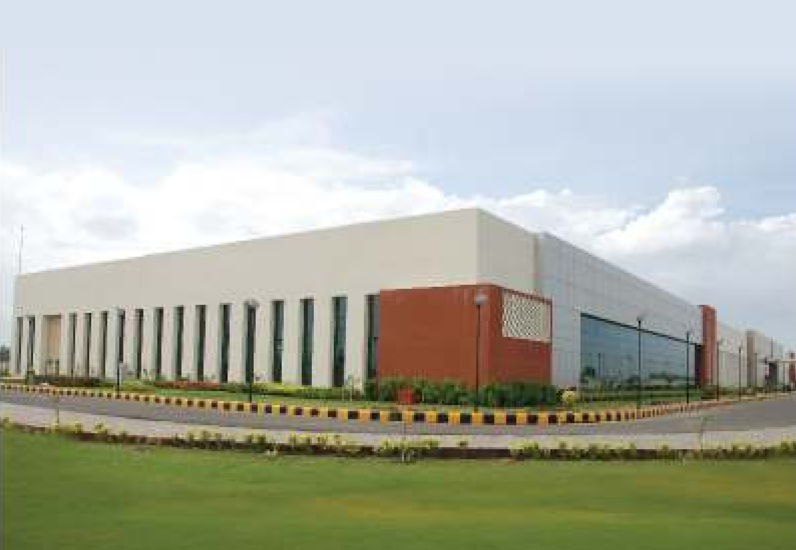
Switchgear Factory, Vadodara
