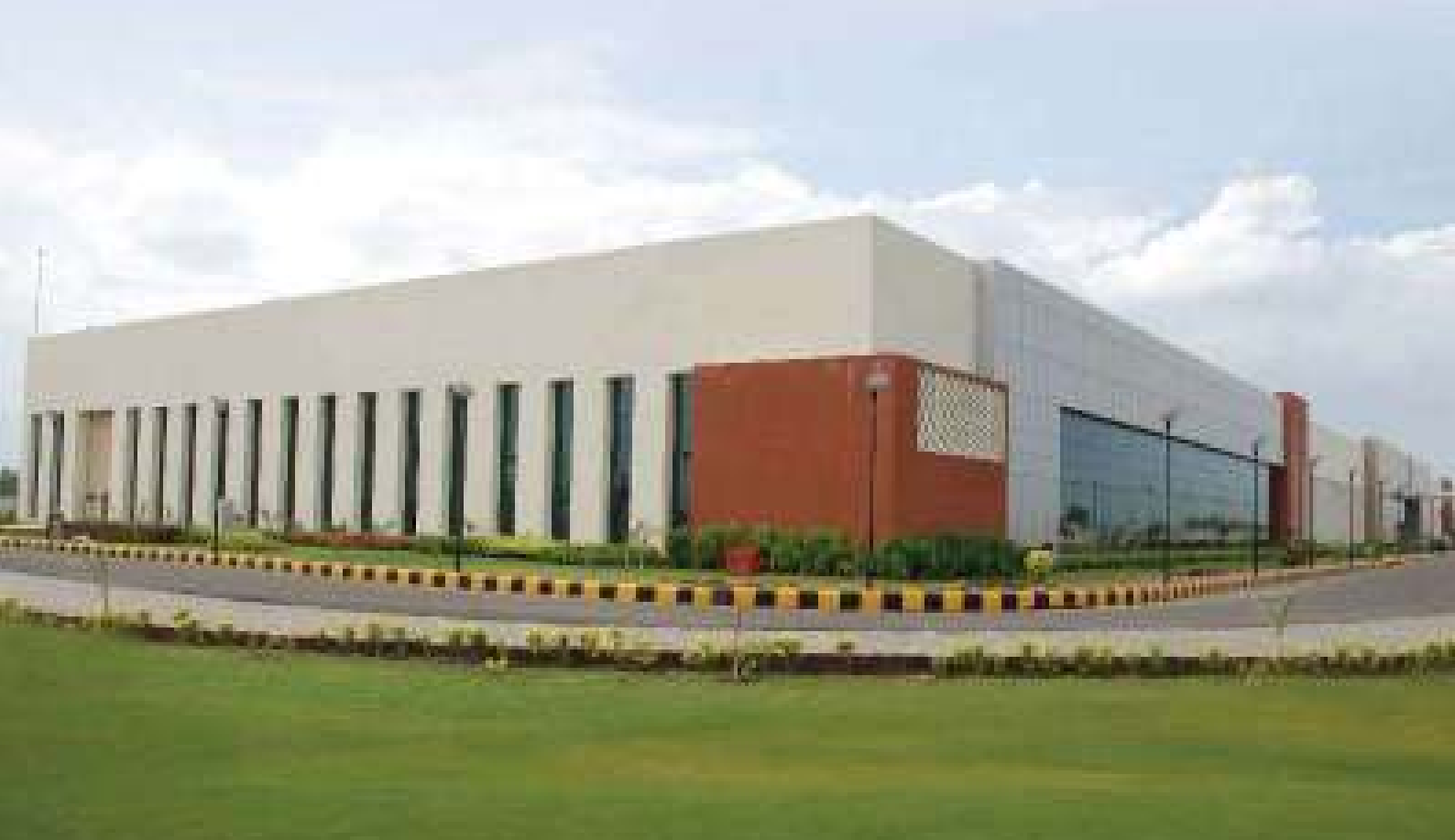
Switchgear Factory, Vadodara
