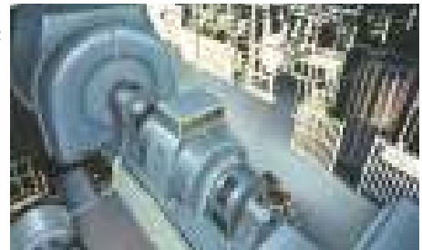
Short-circuit test generator No.1
