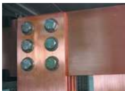
^ Connection on 120 x 10 bars (4000 A)
