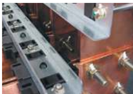
^ Connection on 120 x 10 bars (4000 A)
