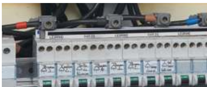
^ Distribution via supply busbars
