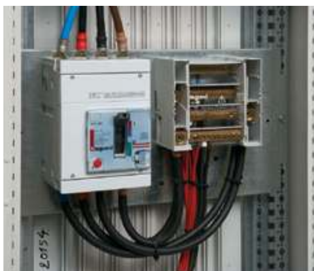
^ For the supply end of medium power distribution panels, the 250 A modular distribution block Cat. No. 048 77 can also be fixed on a plate
