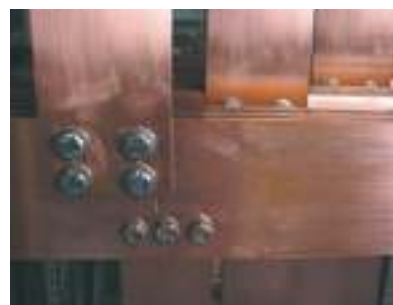
^ Double connection: 100 x 10 bars (3200 A) and 80 x 10 bars (2500 A) on common 120 x 10 bars
