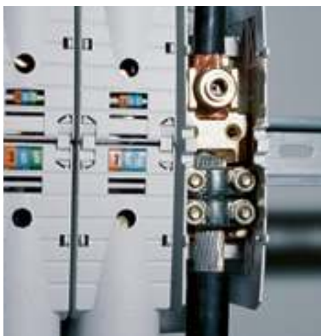
< Alumin./copper direct connection
