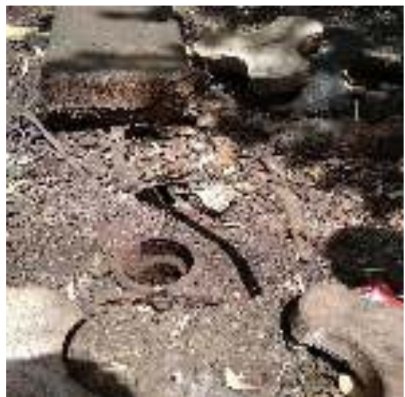
Figure 18. Improper maintenance of earth pits
