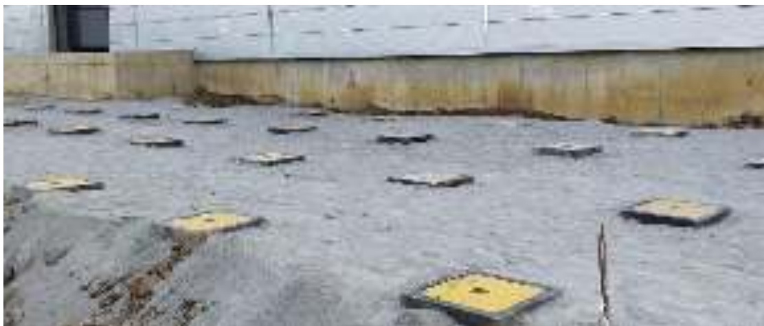
Figure 35. Multiple earth electrodes in parallel connection
