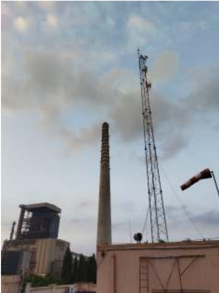
Figure 43. Telecommunication tower in building
