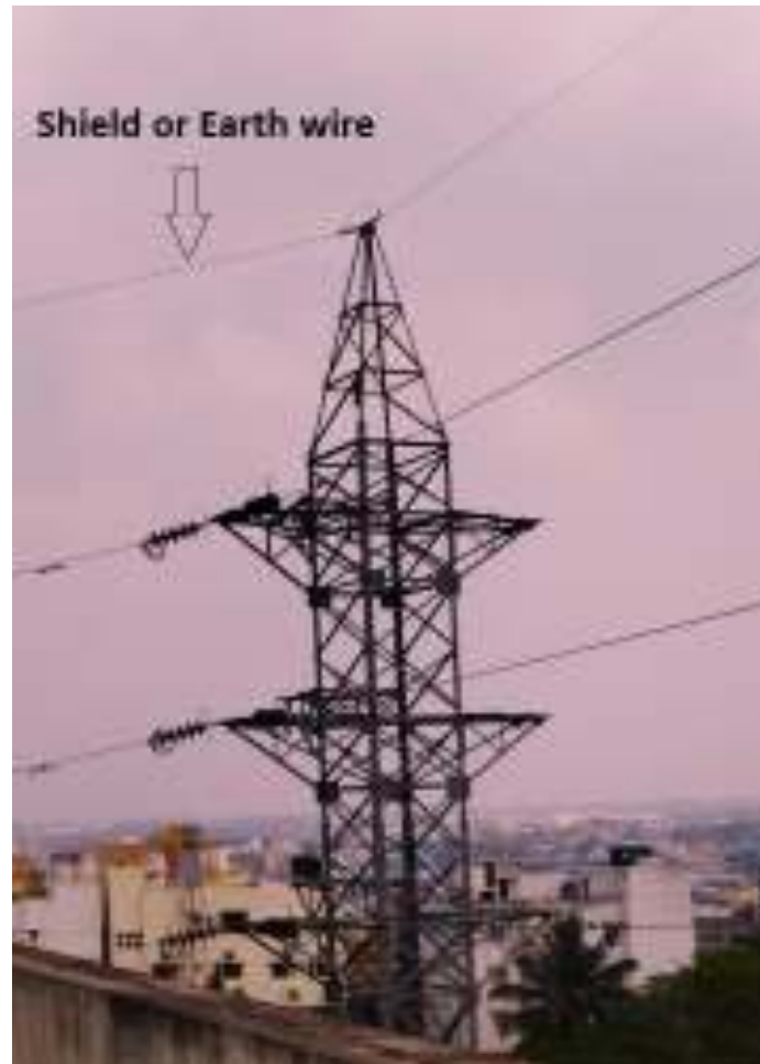
Figure 34. Shield or earth wires in transmission lines
