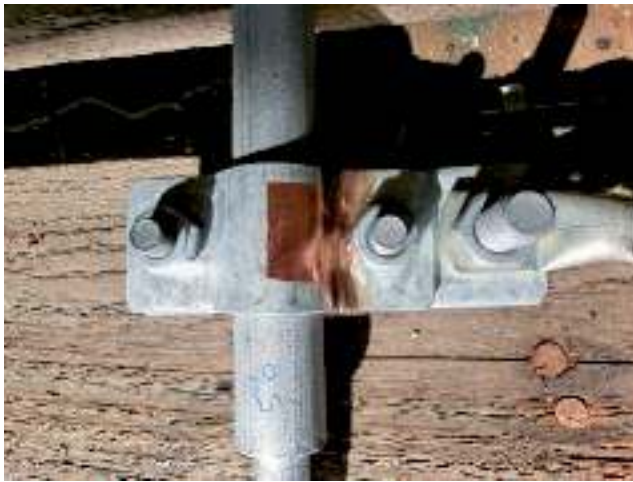
Short-circuit current test on earth rod terminal
