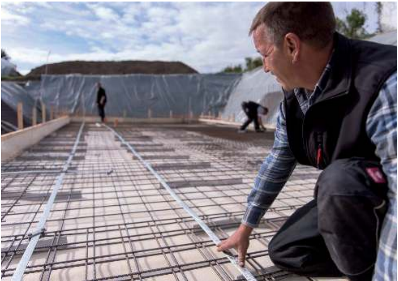
Installing a foundation earth electrode
