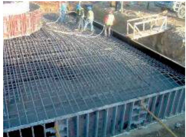
Working on an earthing system of a wind power plant
