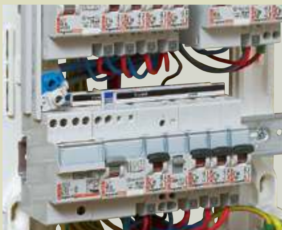
The combination of splitter busbar and vertical prong-type supply busbar enables supply via a voltage surge protector protected by the RCCB and beyond the row...
