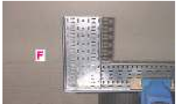
Figure 88: Construct a flat Bend 90° (F)
