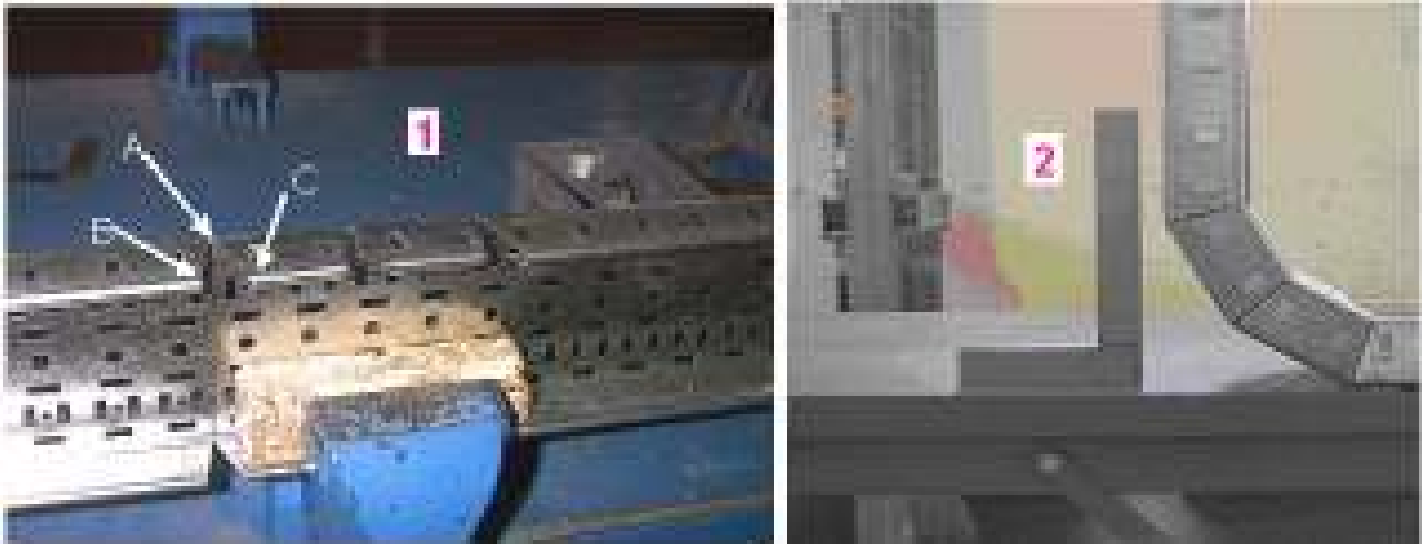
Figure 96: Construct a 90° internal bend
