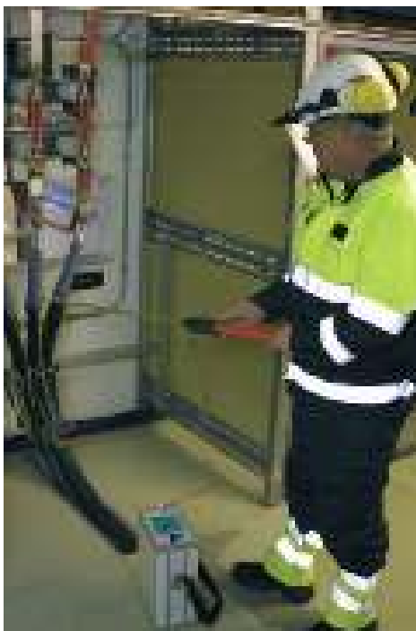
Figure 151: On-line testing of HV cable heads
