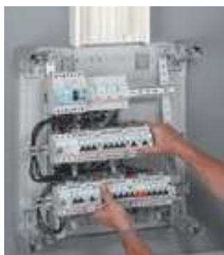
^ When the side panels have been removed, the wiring is fully accessible
