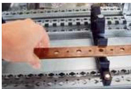
^ Flat bars in cable sleeve
