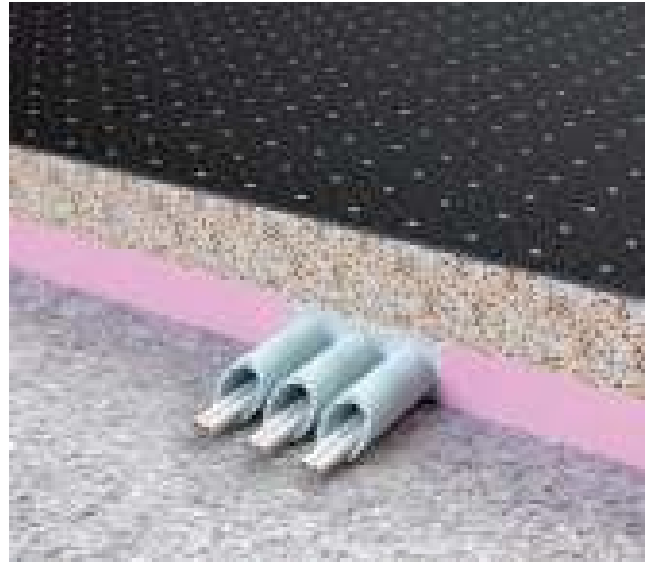
Routing under the screed
