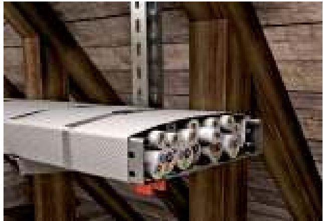
Bandaged cable support systems in areas with many combustible materials
