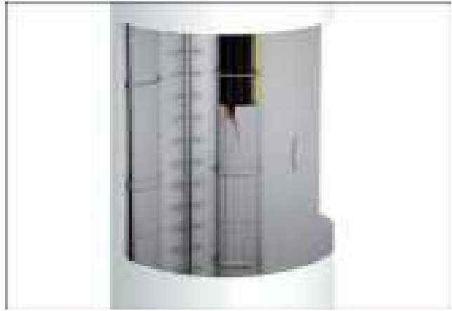
Bandaged rising section in the tower of a wind power plant
