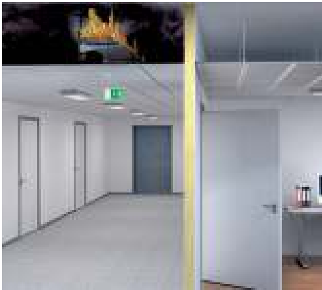
F30 ceiling with fire from above
