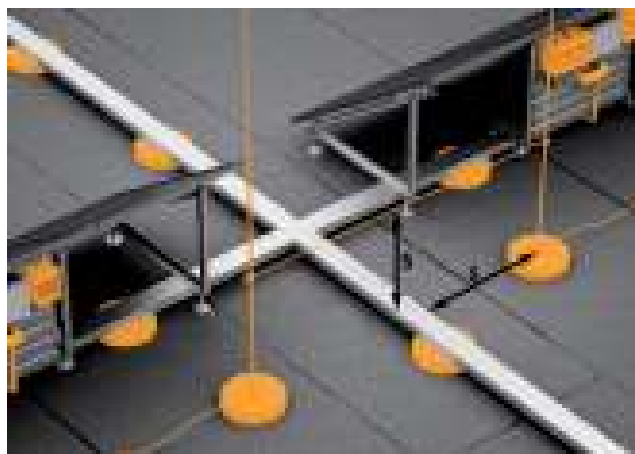
PV system in the protection area of the air-termination system situated at a separation distance of s
