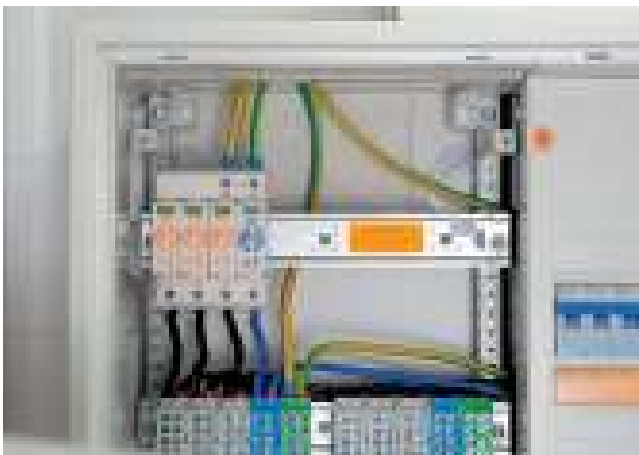
Mounting of the type 1+2 V50 combination arrester in the upper meter connection compartment
