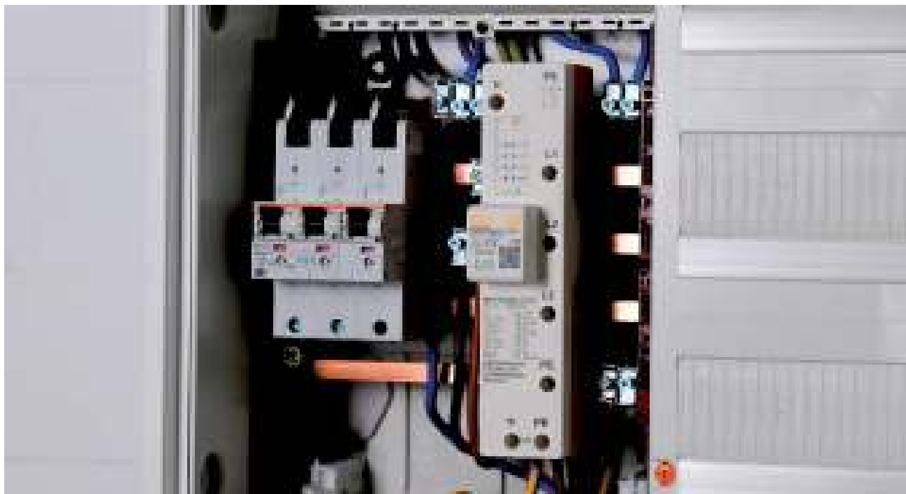
Type 1+2 combination arrester MCF...NAR on the 40-mm busbar in mains-side connection compartment
