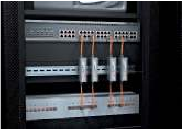
Suggested protection for switch with patch panel. The surge protection devices are earthed via the DIN rail.
