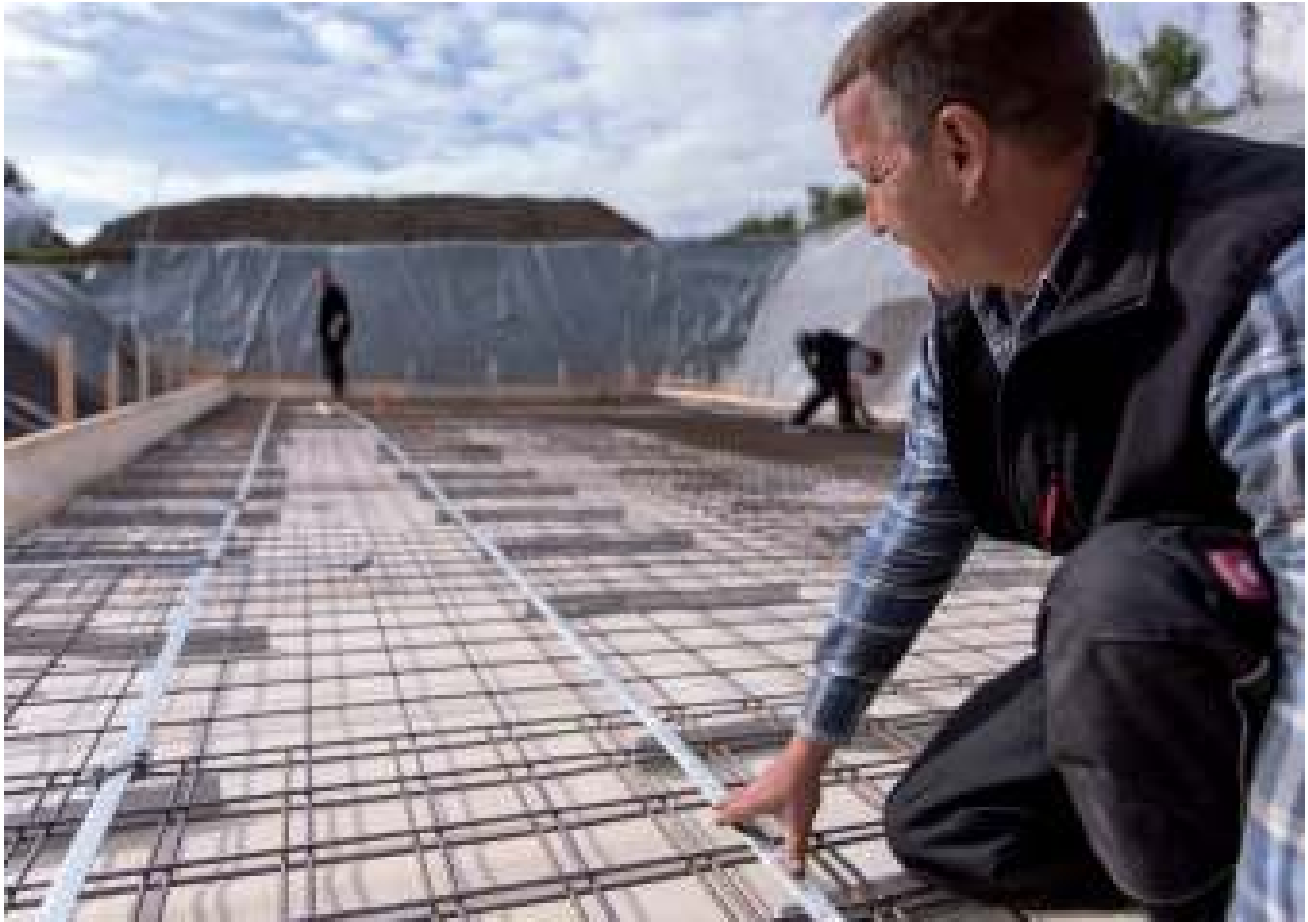
Installing a foundation earth electrode
