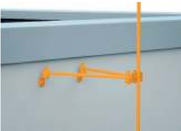
Example: air-termination system with Iso-combination set for V fastening
