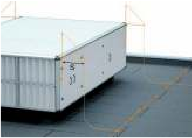
Example: air-termination system with Iso-combination set for triangular fastening
