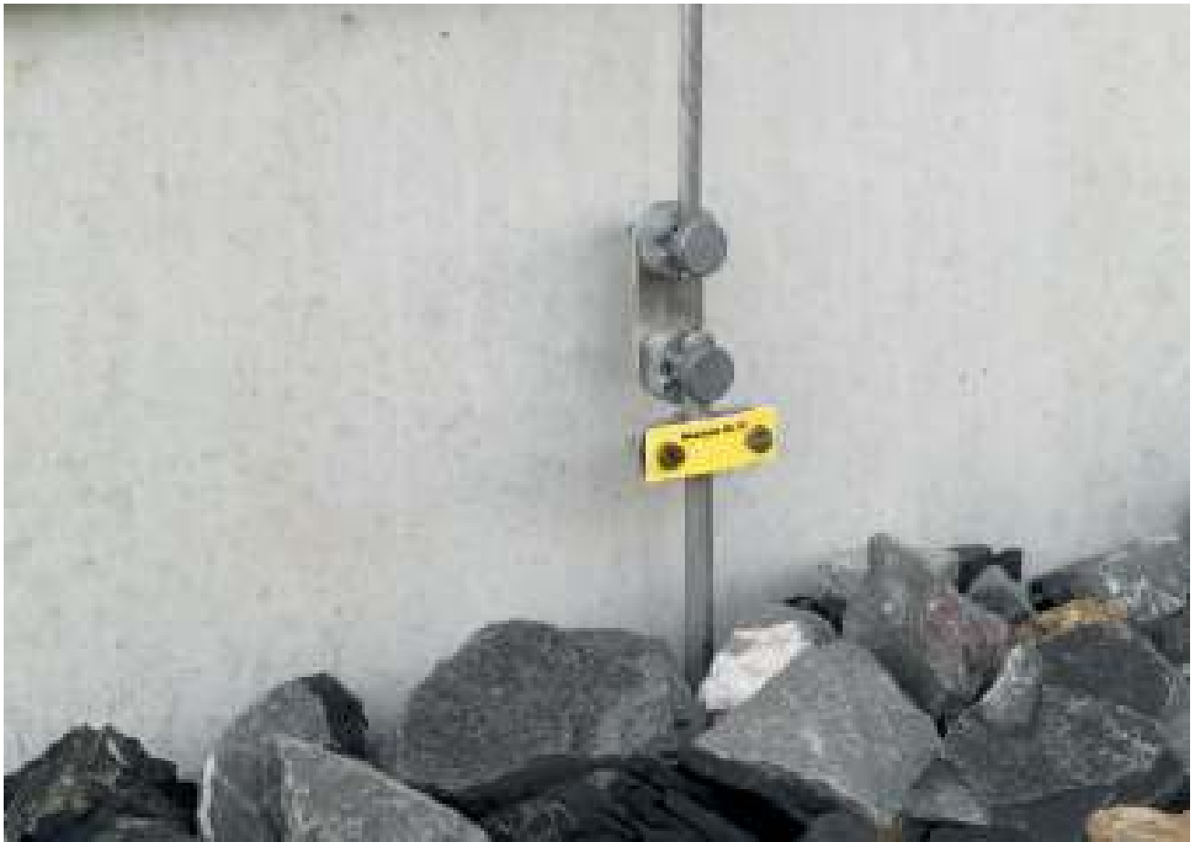
Separation point on a metal facade
