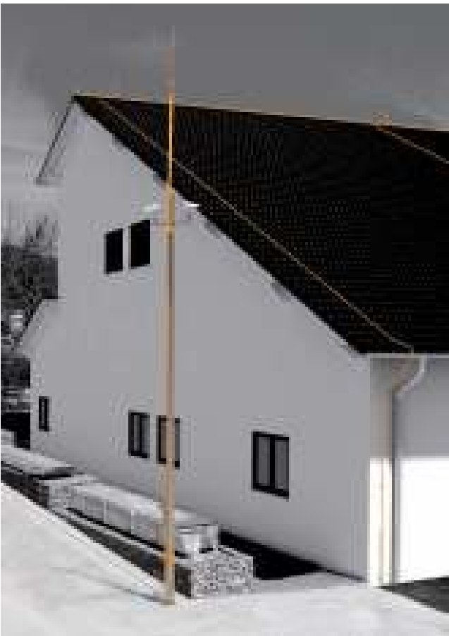
CCTV cameras with isCon® conductor
