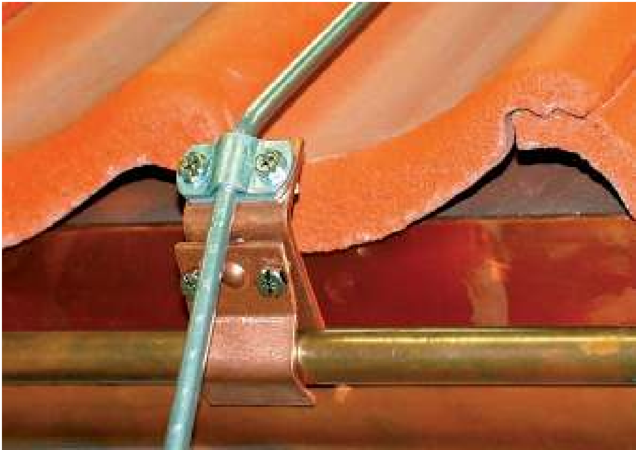
Bi-metal roof gutter clamp (aluminium round conductor and copper roof gutter)
