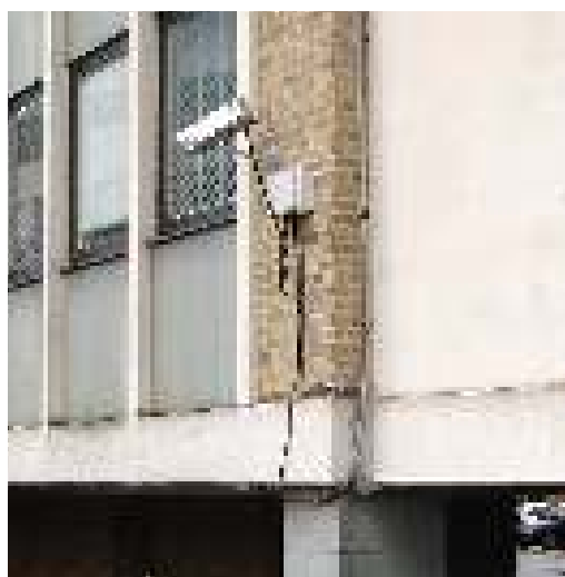
Figure 65. Conventional down-conductor separation distance problem.
