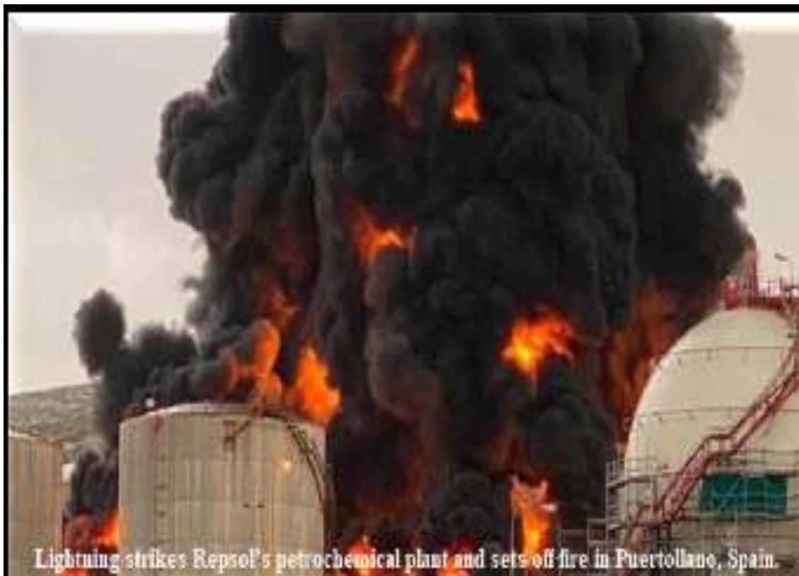
Figure 39. Explosion in tank farm
