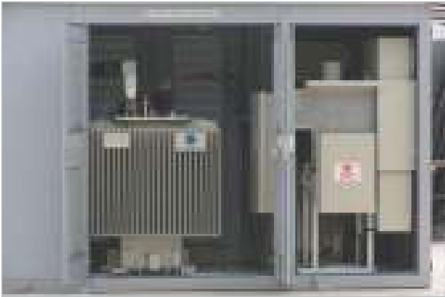
Figure 3.4: Transformer Compartment
