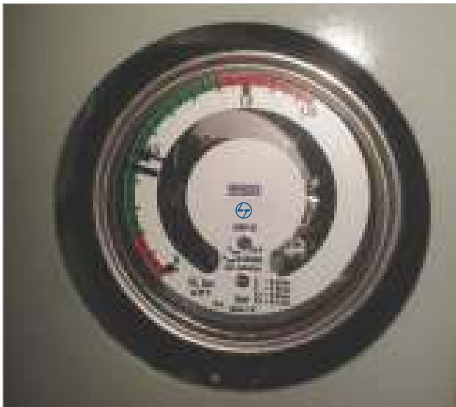
Figure 3.7.1: Gas Pressure Indicator
