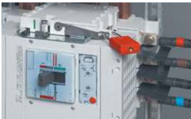
^ Draw-out DPX 630 immobilised using padlocks
