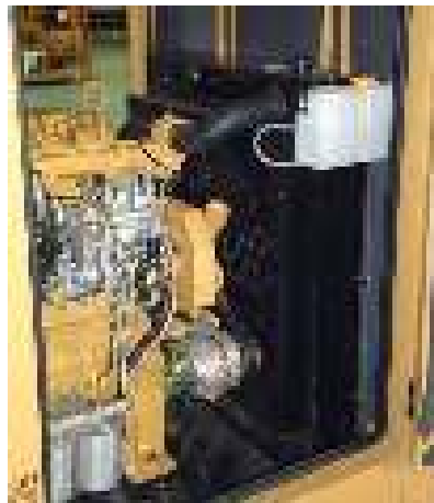
Fig. B1.4 Radiator Cooling System
