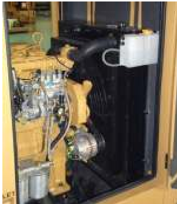
Fig. B1.4 Radiator Cooling System
