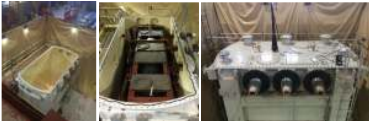
Figure 3.8 - Cleaned Tank, Core/Windings Back in Tank and Sealed Tank
