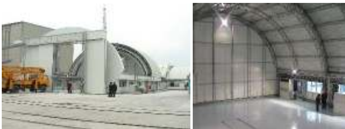
Figure 3.26 - left: Repair facility outside view with open roof top; right: Repair facility inside view with air conditioning device and heater
