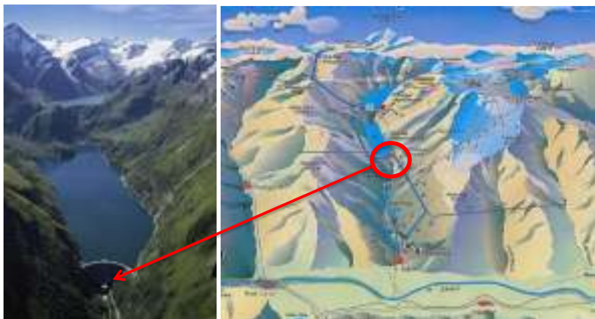
Figure 2.26 - Kaprun Water Storage Power Plant Limberg (Source: German newspaper Augsburger Allgemeine)
