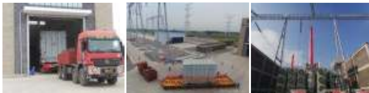
Figure 2.50 - Transportation and installation in substation of on-site assembly transformer
