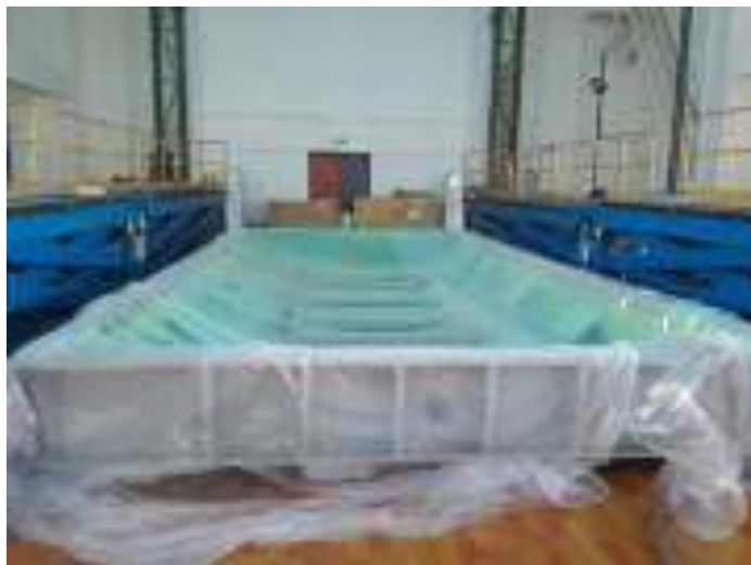
(a) Lower oil tank into position
