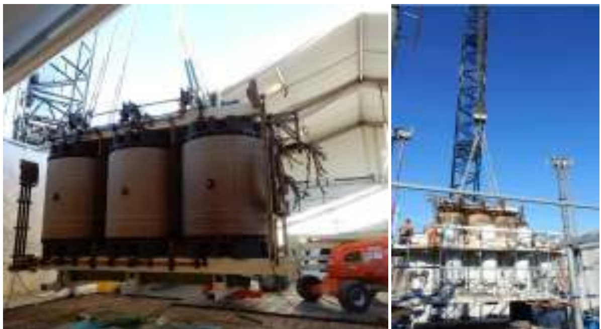
Figure 3.16 - Heavy Crane Lift of Repaired Core/Windings
