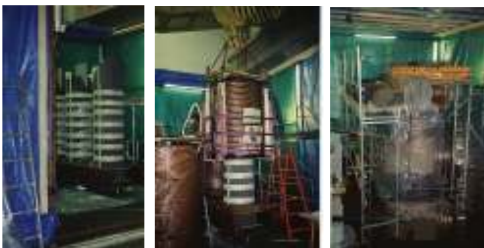
Figure 2.29 - left: Core after upper yoke and clamping removal inside the tent; middle: Winding block fitting to the core; right: Upper yoke stacking
