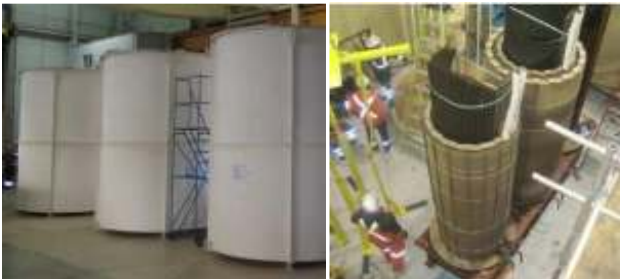
Figure 3.6 - New Winding Shipping Containers and Installation of New Windings
