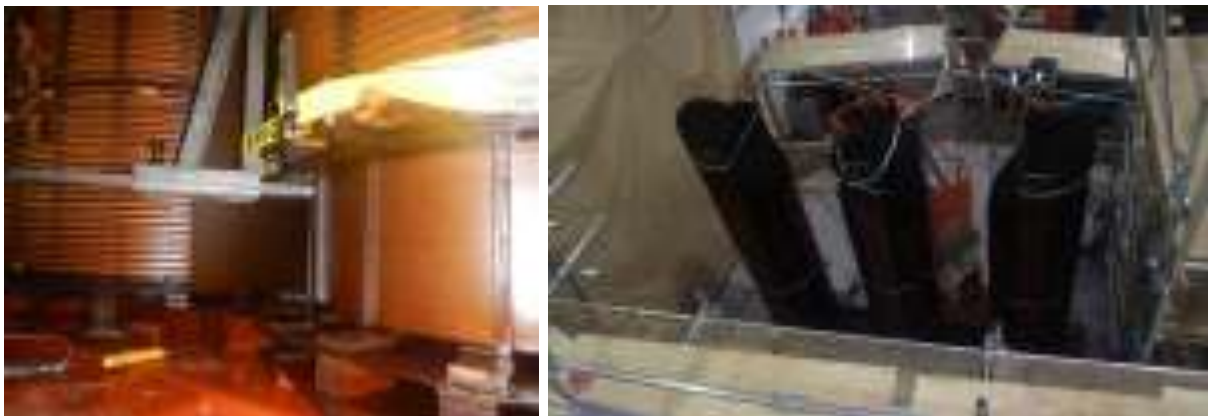
Figure 3.5 - Removal of Windings
