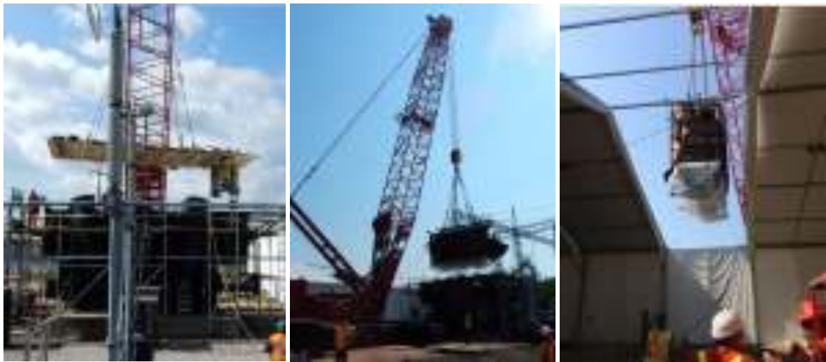
Figure 3.12 - Removal of the Cover and Removal of the Core/Windings from the Tank
