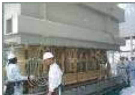
(j) Insertion of middle tank
