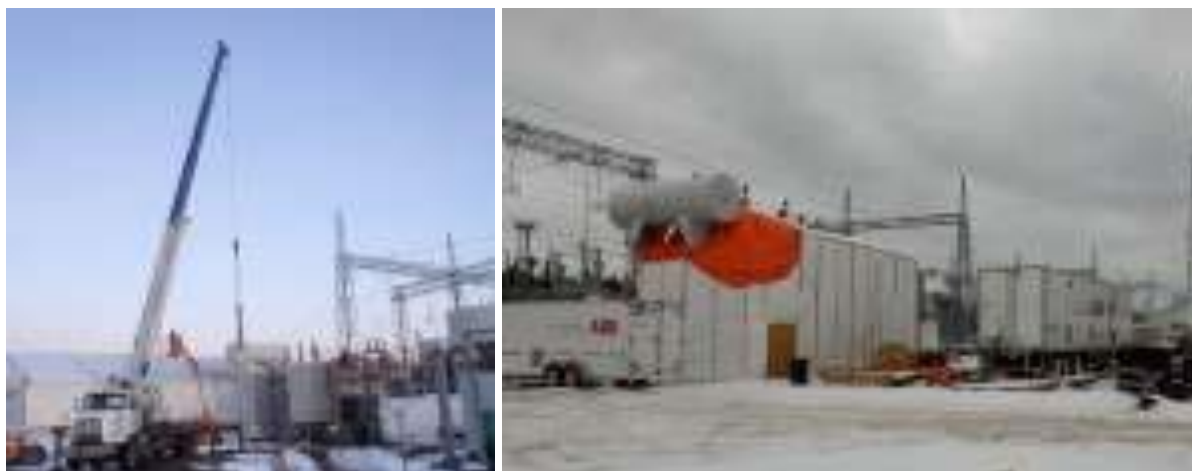
Figure 3.17 - Installation of Bushings, LFH Dryout (hoarding required due to cold weather)
