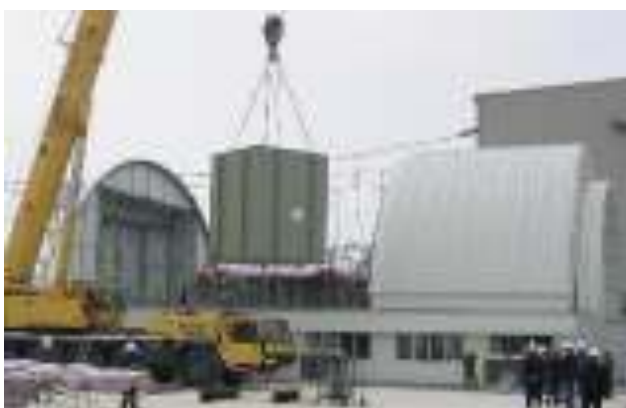
Figure 3.29 - left: Drawing of winding block shipment tank; middle: Lifting of winding block tank into repair facility; right: Removal of damaged limb while new winding block stand beside for replacement
