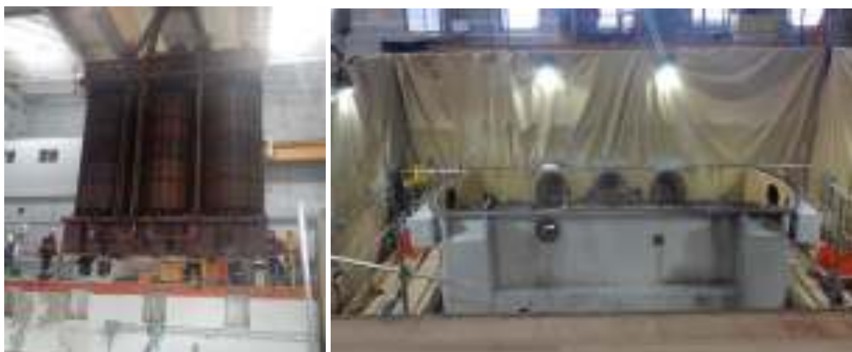
Figure 3.3 - Core/Windings Being Removed from the Tank
