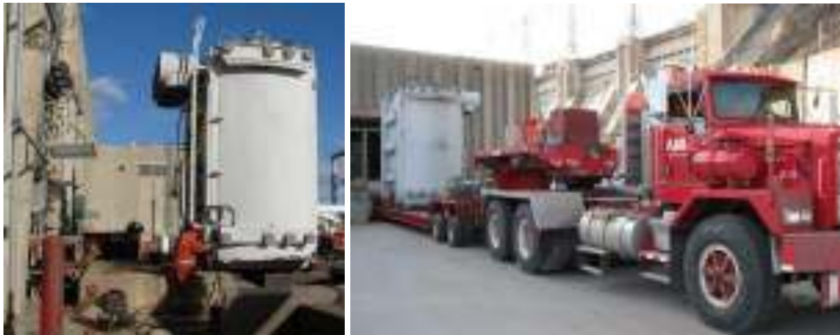
Figure 3.1 - Transformer Being Moved from Pad to Turbine Hall
