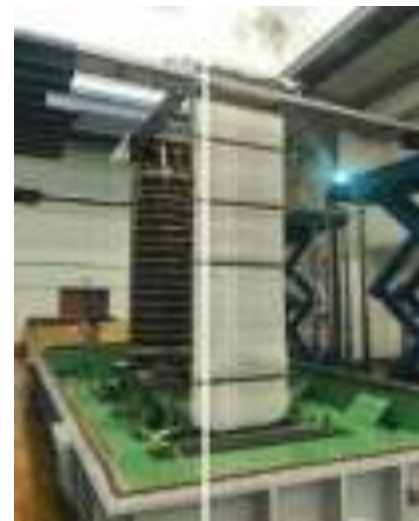
(b) Assembly of No.2 U-shaped core frame
