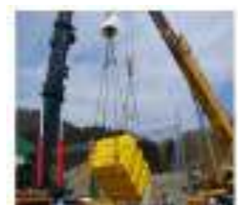
(f) Lifting of core by 2 cranes (400 t and 100 t)
