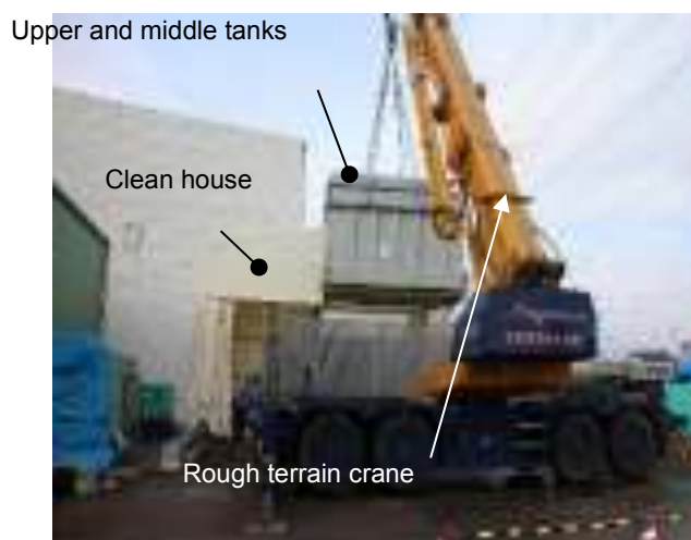
Figure 3.38 - Lifting upper and middle tanks
