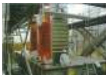
(g) Installation of core by crane
