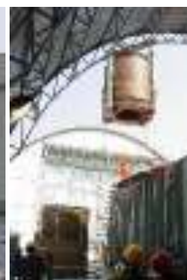
Figure 3.29 - left: Drawing of winding block shipment tank; middle: Lifting of winding block tank into repair facility; right: Removal of damaged limb while new winding block stand beside for replacement
