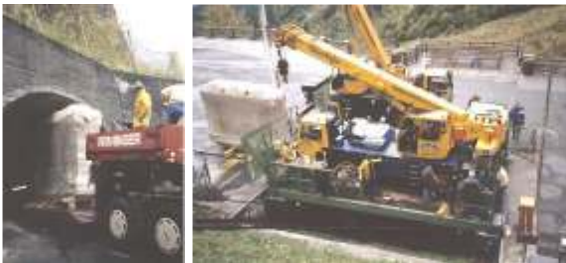
Figure 2.27 - left: Road transportation of core with special low road vehicle; right: Loading of core on elevator at mountain valley station
