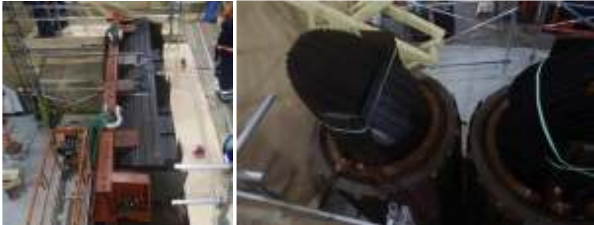
Figure 3.4 - Removal of the Top Yoke of the Core
