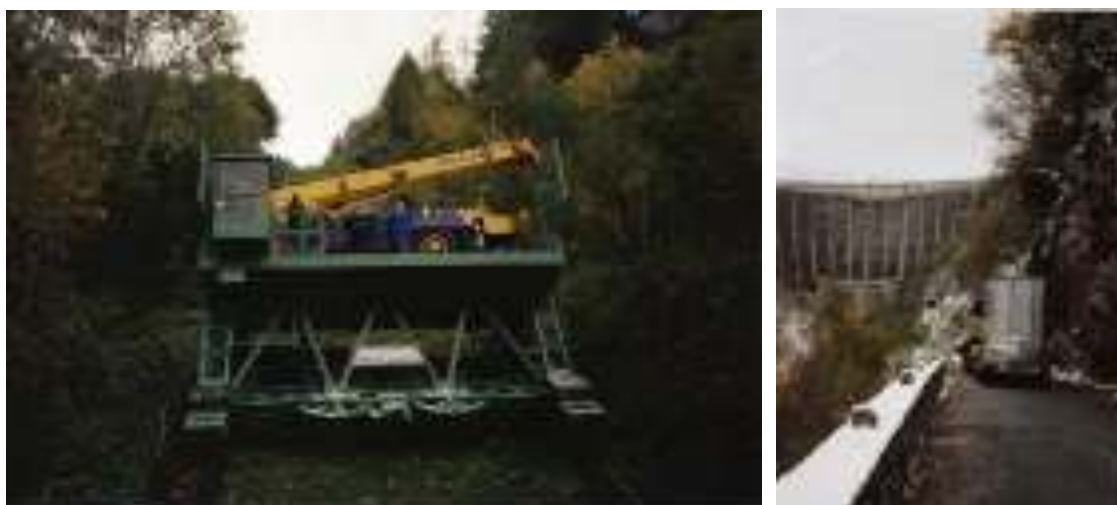
Figure 2.28 - left: Mountain elevator to lift devices, core and tank including winding blocks to the middle station Lärchenwald of Kaprun mountain; right: transportation from elevator to power station via road transport vehicle, here: tank transportation including winding blocks
