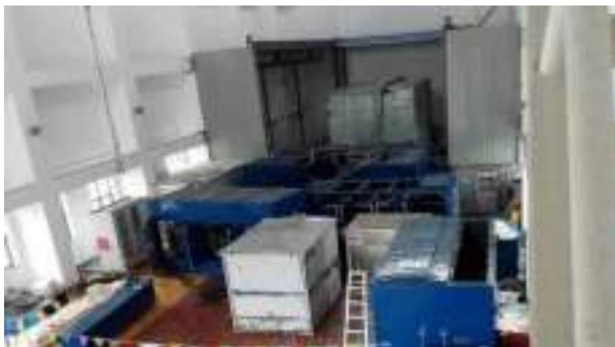
Figure 2.49 - Kerosene vapour phase drying treatment for transformers
