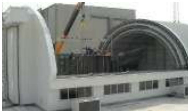
Figure 3.28 - left: Sketch of disassembly; right: Photo taken during upper clamping arrangement disassembly
