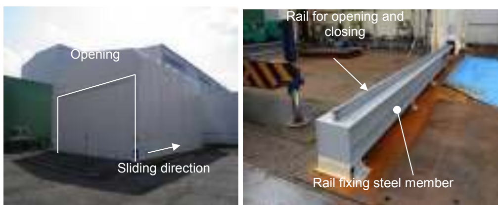
Figure 3.40 - Clean house installation states
