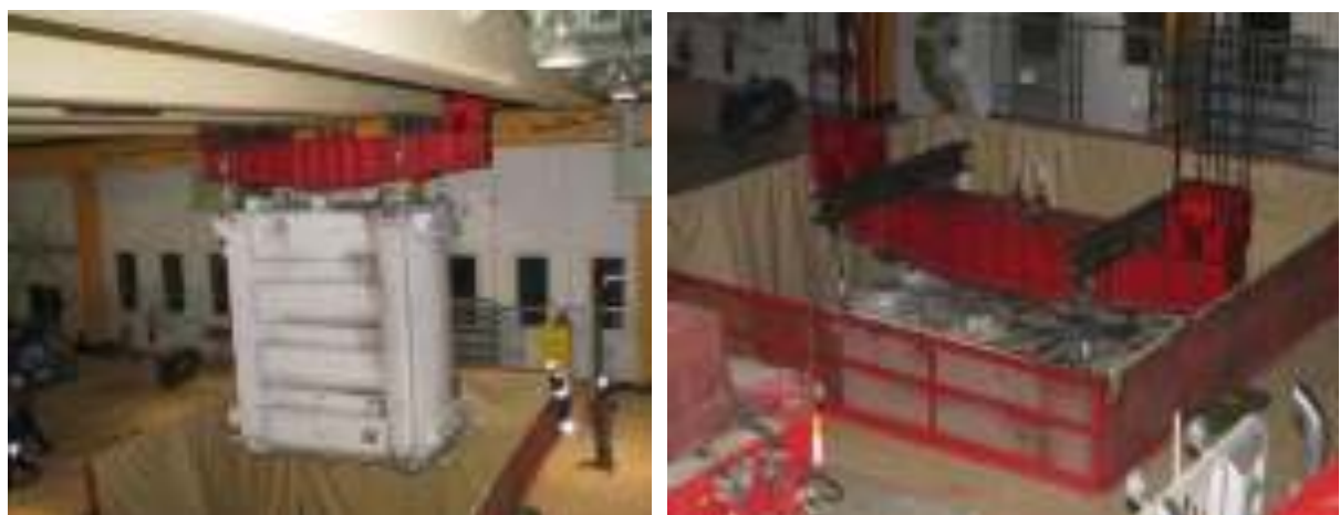
Figure 3.2 - Transformer Being Moved into Turbine Hall Pit with Overhead Crane
