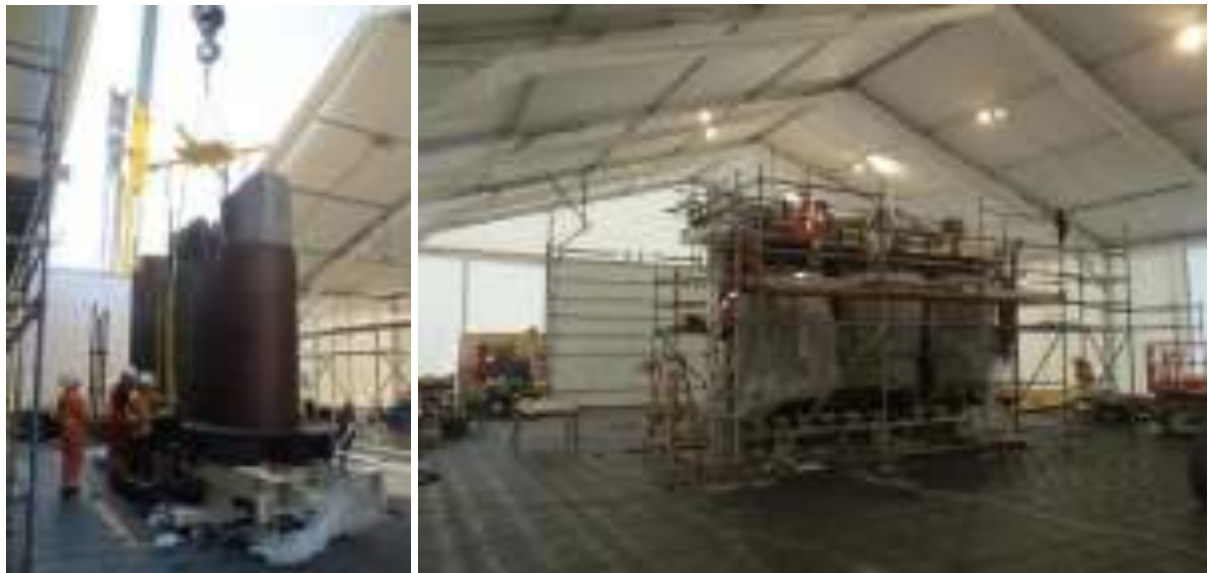
Figure 3.14 - Installation of New Windings and Core/Windings being worked on
