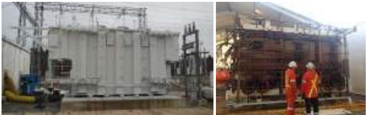
Figure 3.15 - Painted Tank (done on pad) and Completed Core/Windings
