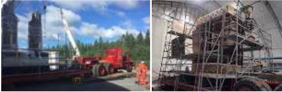
Figure 3.24 - Transformer New Winding Installation and Cleats & Leads Work
