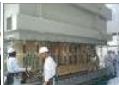
(f) Insertion of middle tank
