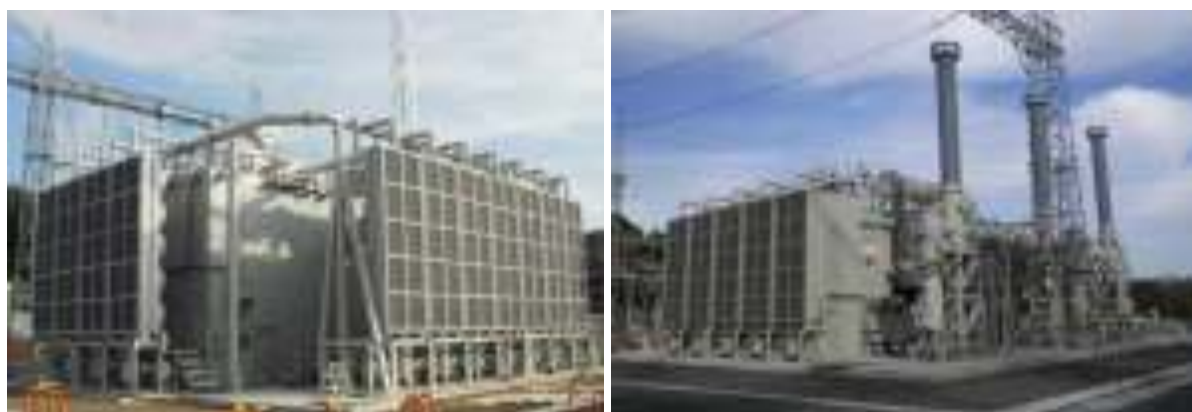
Figure 2.17 - On-site assembly transformer after completing its installation (500 kV - 1 000 MVA)
