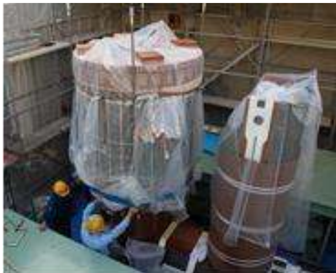
Figure 3.42 - Winding refurbishment work in clean house
