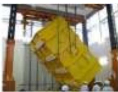
(b) Erecting of core tank by lifter
