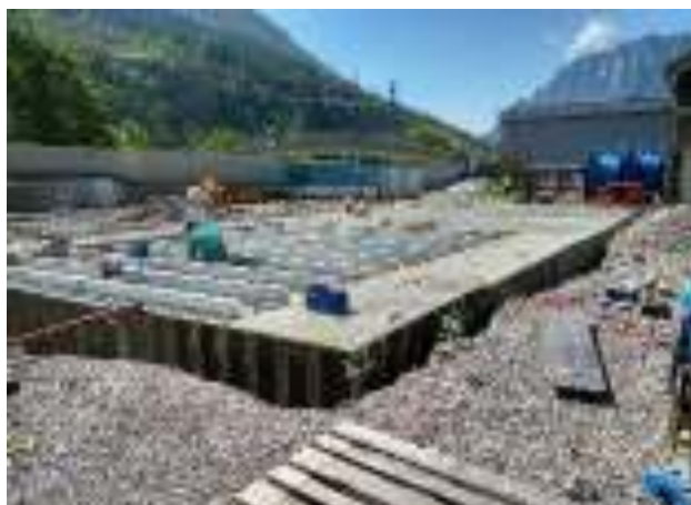
(b) Foundation of the transformer
