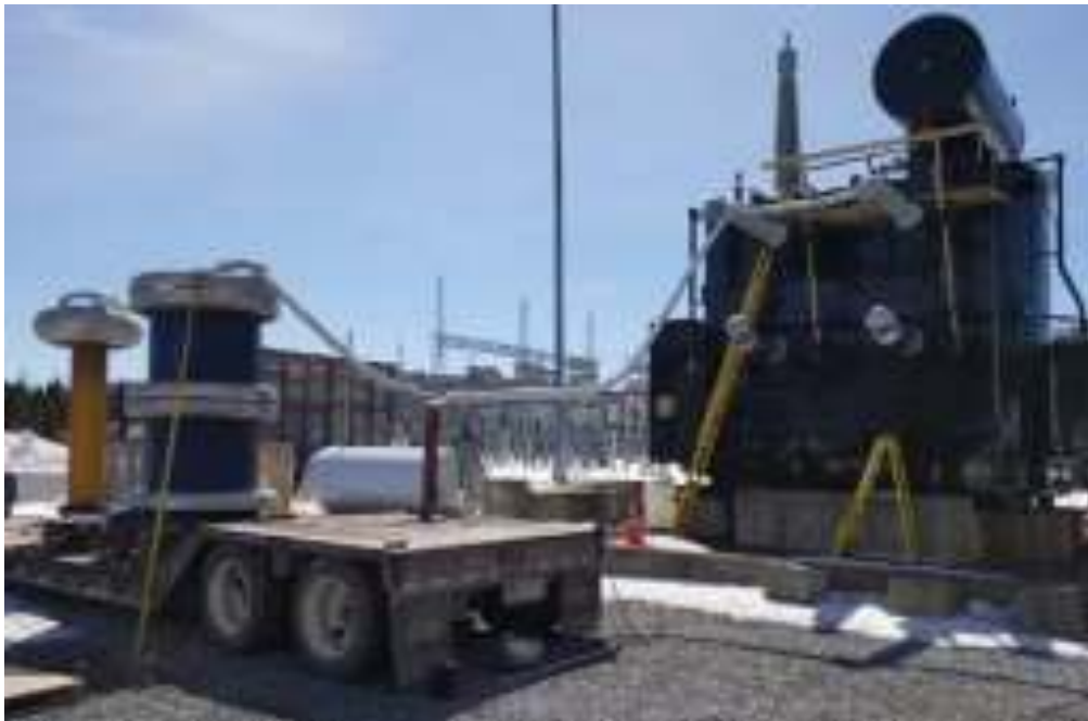
Figure 3.25 - DC HV Testing
