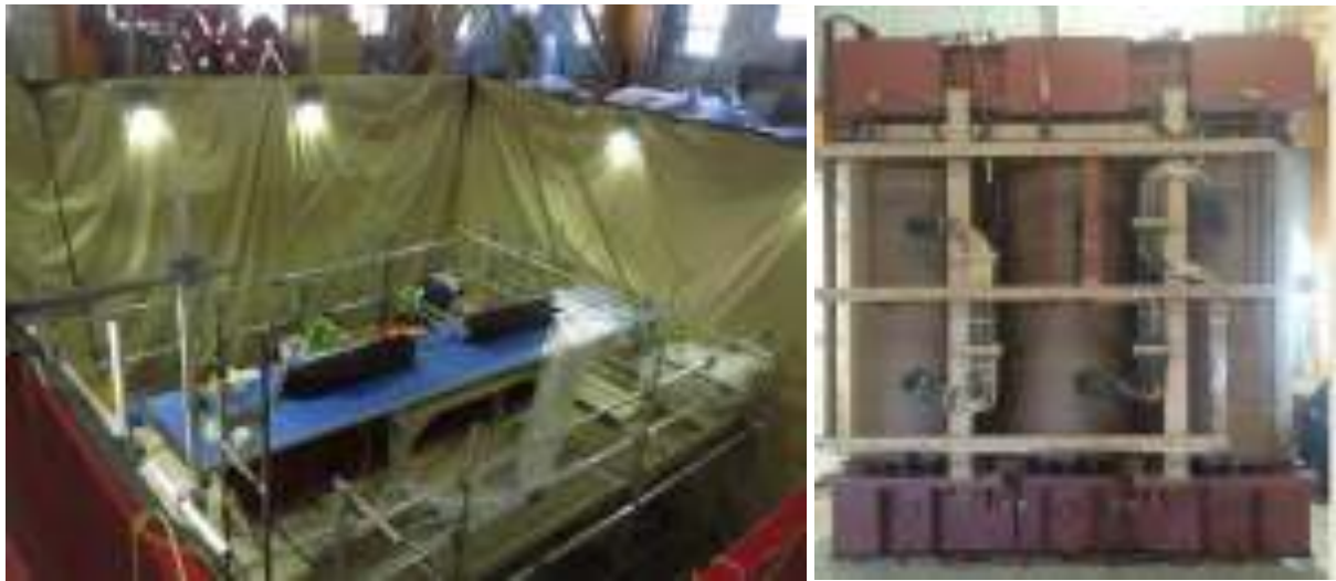
Figure 3.7 - Re-installation of Top Yoke of Core and Finished Core/Windings
