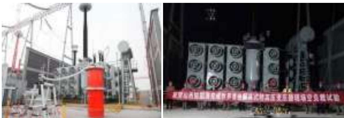
Figure 2.51 - Acceptance test of on-site assembly transformer
