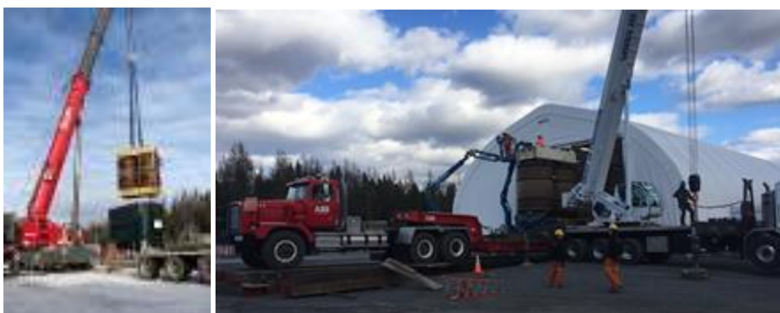
Figure 3.23 - Transformer Un-tanking
