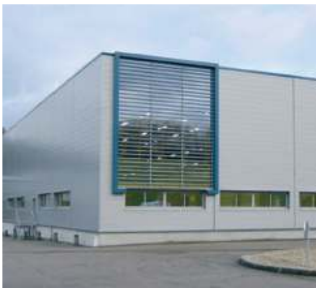
^ Controlled solar protection on an industrial building
