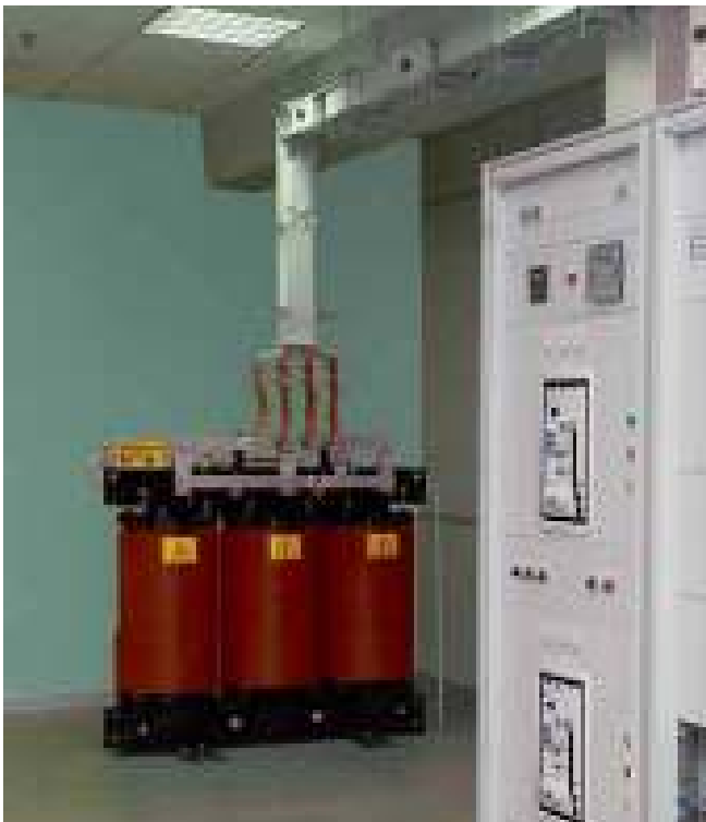
< Link between the transformer and the main LV distribution board by Legrand high power prefabricated busbar system
