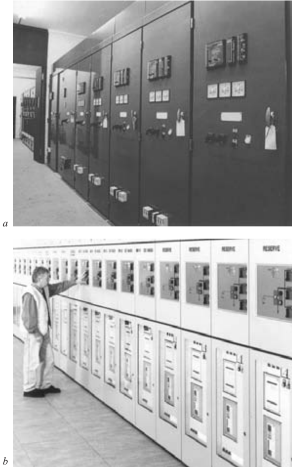
Figure 9.5 Examples of vacuum switchgear
