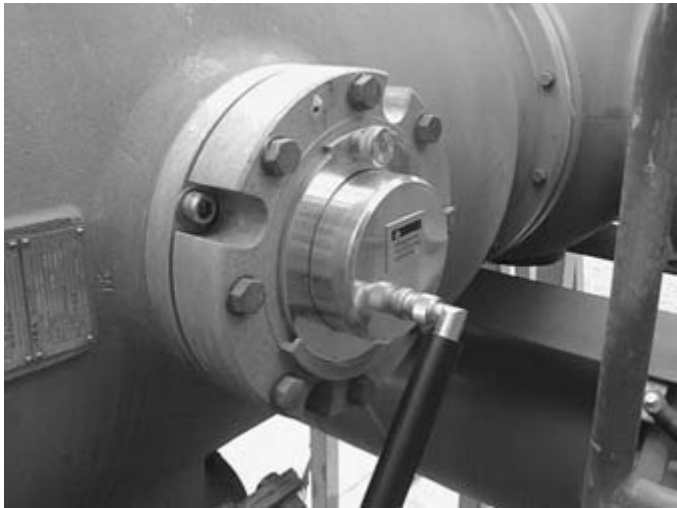
Figure 2.15 An external window coupler on a 500 kV GIS
