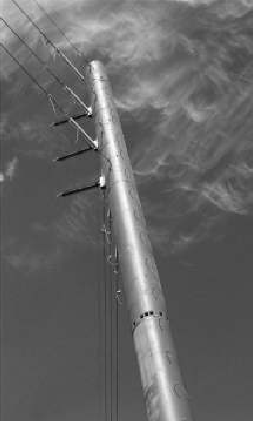
Figure 1.6 Prestressed Concrete Pole.
