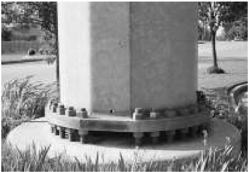
Figure 1.4d Drilled Shaft Foundation for a Steel Transmission Pole.
