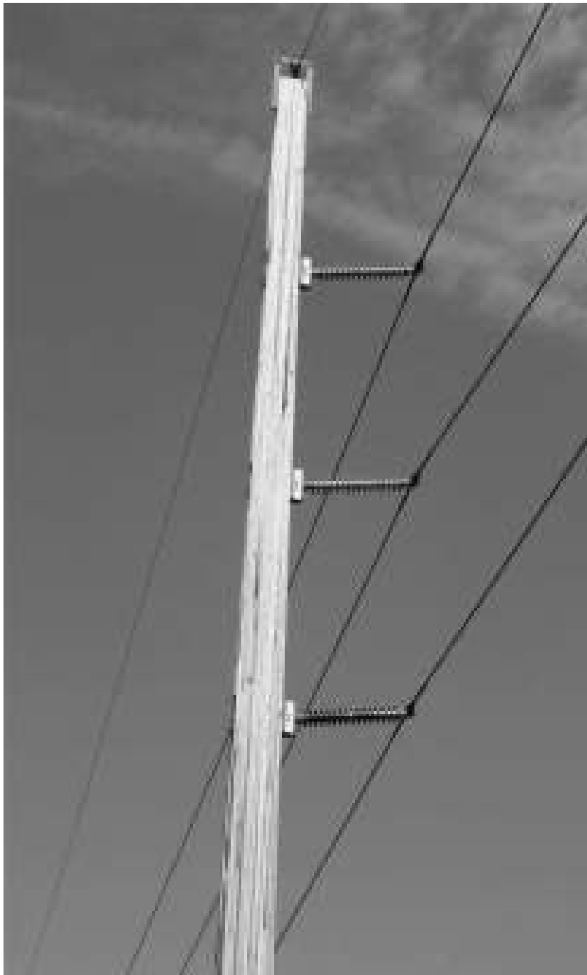
Figure 1.7 Laminated Wood Pole.
