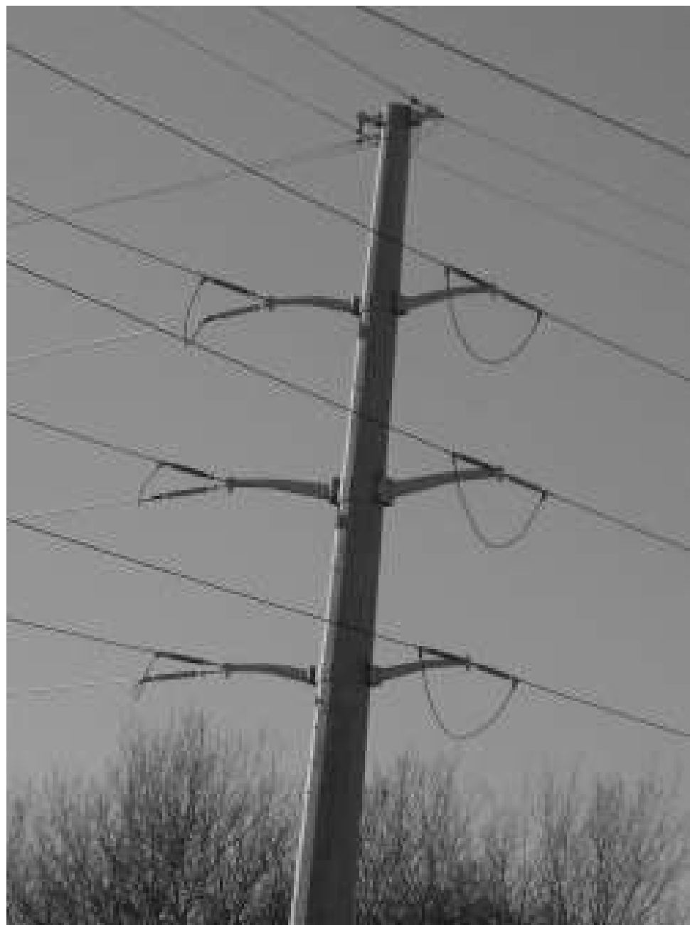
Figure 1.4b Steel Pole Deadend – Tangent and 90 degrees.
