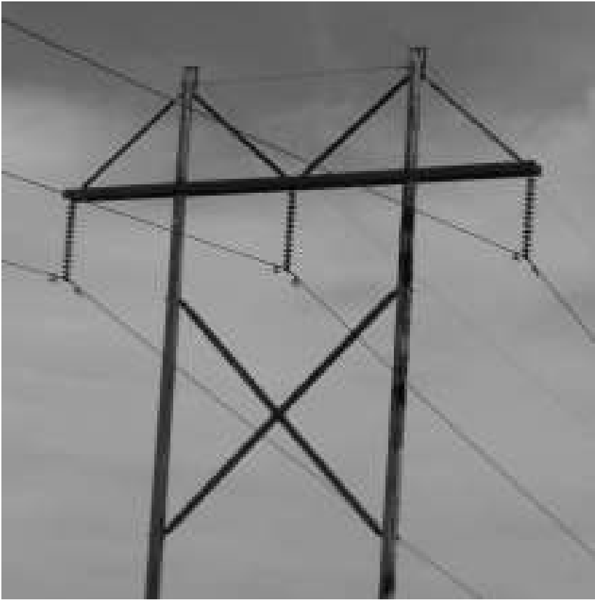
Figure 1.3a Wood H-Frame.
