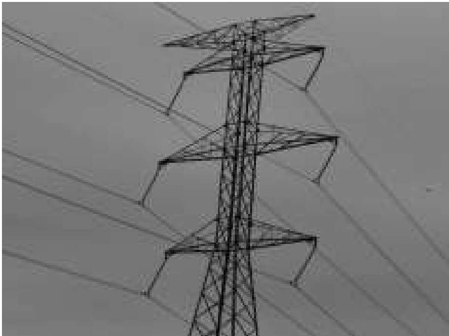
Figure 1.5 Lattice Tower.
