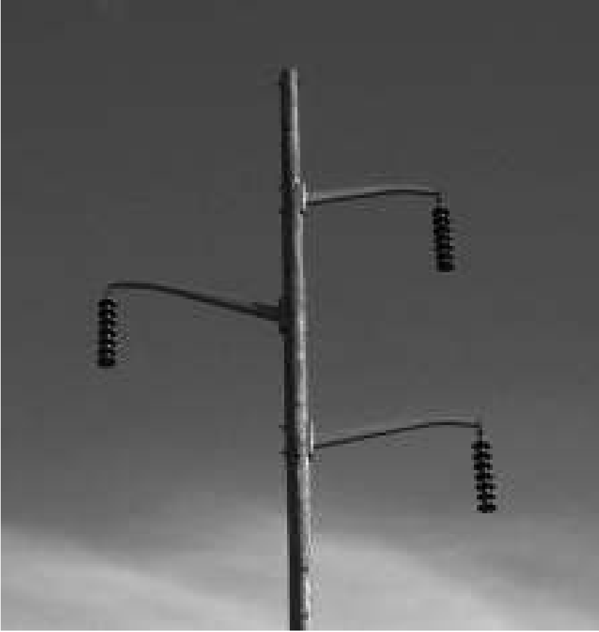
Figure 1.3b Wood Pole with Steel Davit Arms.
