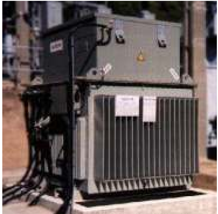
Figure 139: Petersen compensation coil (Alstom)
