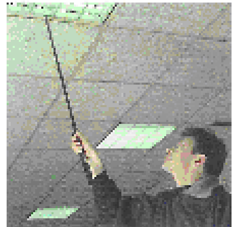
Figure 50: Continuity check with contact stick
