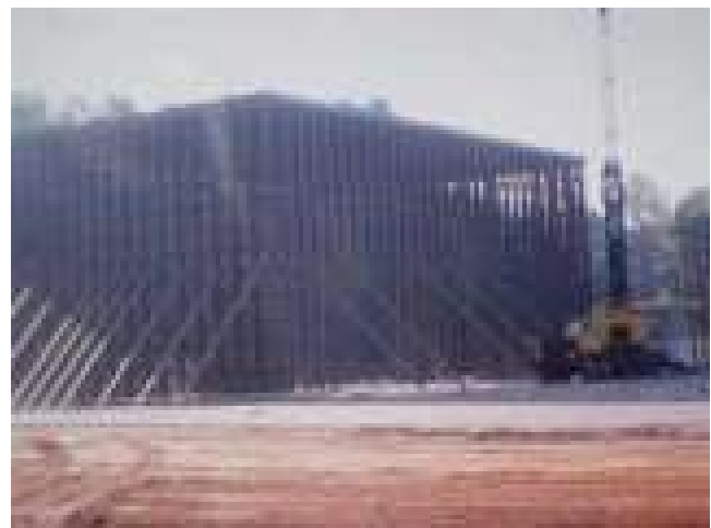
Figure 26: Faraday cage in construction (ammunition depot...)
