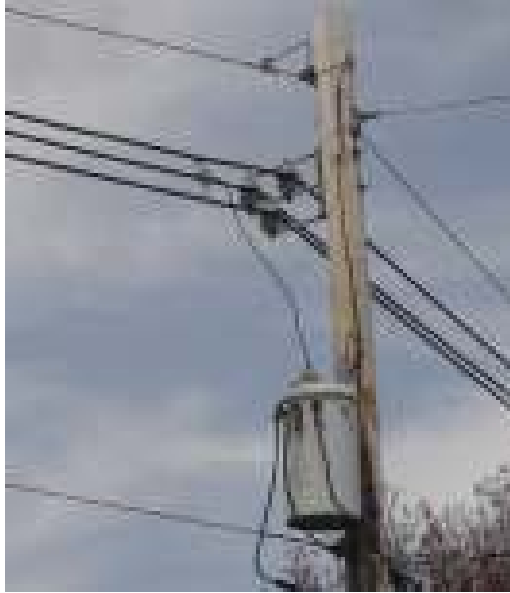
Figure 9.15 Unfused CSP on a mainline.
