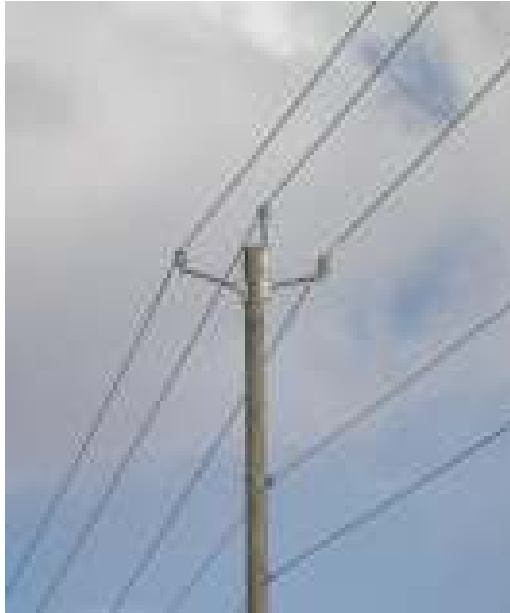
Figure 2.1 Three-phase 34.5-kV armless construction with covered wire.
