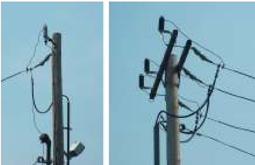
Figure 13.21 Arrester applications with long lead lengths.
