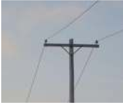
Figure 2.3 Single-phase, 4.8-kV circuit.
