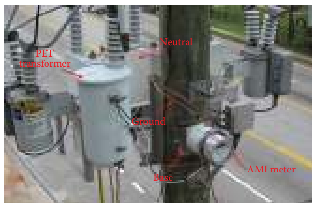
Figure 7.28 Neutral current monitor using AMI. (Courtesy of Georgia Power.)
