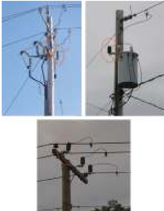
Figure 13.12 Example of arrester applications.
