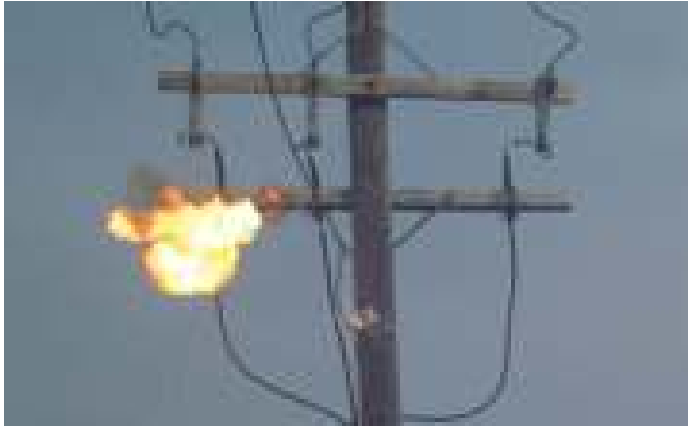
Figure 9.3 Example operation of an expulsion fuse during a fault. (Courtesy of the Long Island Power Authority.)
