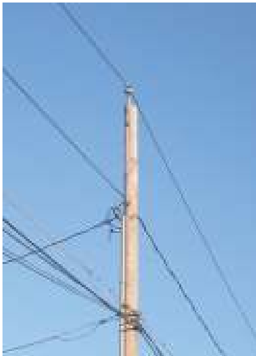
Figure 2.2 Single-phase circuit, 7.2 kV line-to-ground.
