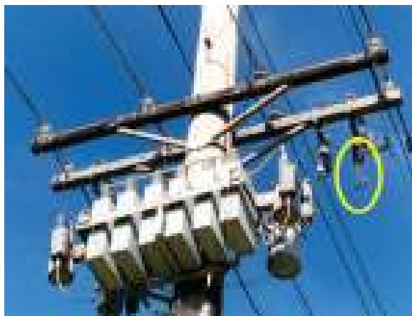
Figure 7.17 Capacitor bank with a blown fuse. (From EPRI 1001691, Improved Reliability of Switched Capacitor Banks and Capacitor Technology , Electric Power Research Institute, Palo Alto, CA, 2002. Copyright 2002. Reprinted with permission.)
