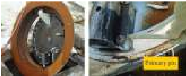
Figure 14.35 Bottom view of a manhole cover with controlled pressure relief. (From EPRI 1015889, Manhole Event Risk Management Strategies: High-Level Overview , Electric Power Research Institute, Palo Alto, CA, 2008. Copyright 2008. Reprinted with permission.)
