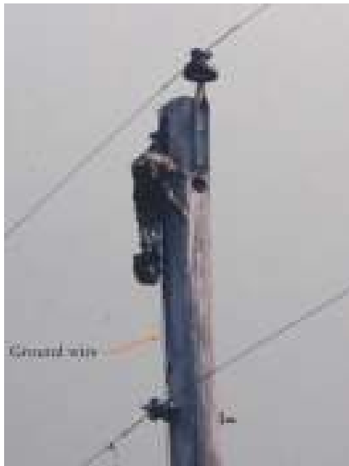
Figure 3.22 Electrocuted cat and the ground wire that made the pole susceptible to animal faults. (Courtesy of Duke Energy.)
