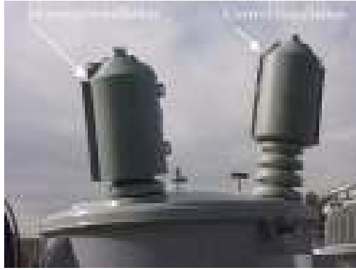
Figure 3.19 Animal guard installation. (From EPRI 1001883, Distribution Wildlife and Pest Control , Electric Power Research Institute, Palo Alto, CA, 2001. Copyright 2001. Reprinted with permission.)
