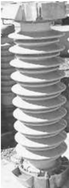
FIGURE 10.8 Post insulators.
