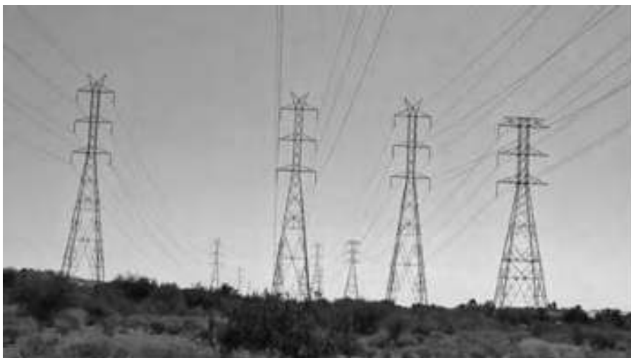
FIGURE 19.3 Transmission line corridor.
