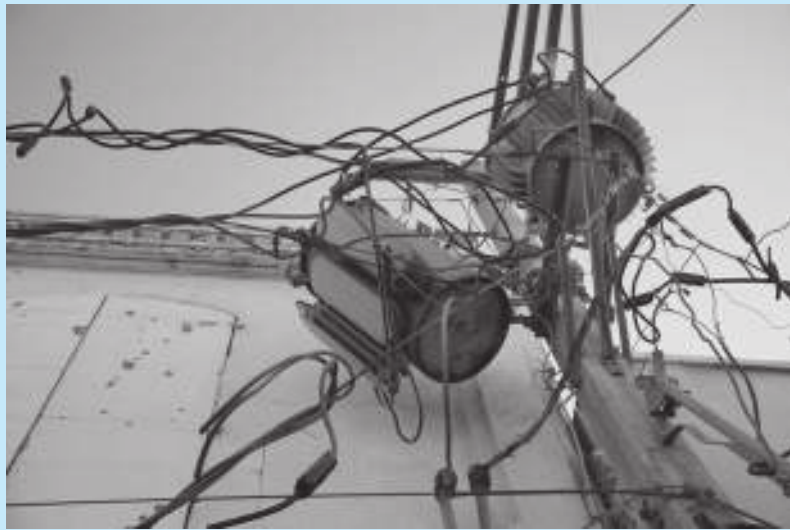
FIGURE 5.19 Destroyed transformer and transmission lines. (Used with permission from © Design Pics Inc. – RM Content/Alamy.)
