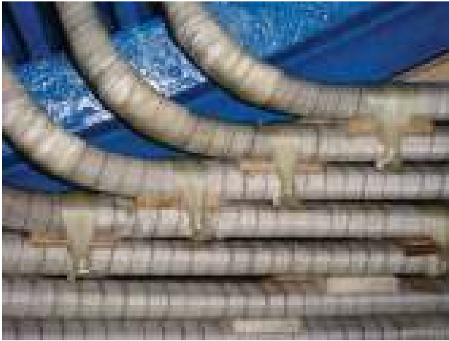
Figure 18.2 Butterfly ties at interbar blocking.
