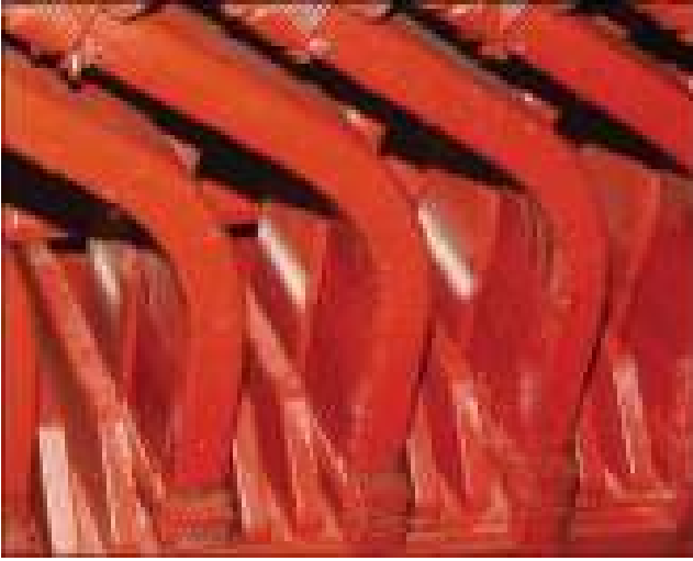
Figure 8.10 Photograph of the end winding area from a hydrogenerator. The white band around some of the coils just outside the slot indicates where the coating overlap area has degraded. Note that the entire stator has been painted with an abrasion resistant coating that makes repair of the overlap problem very difficult.
